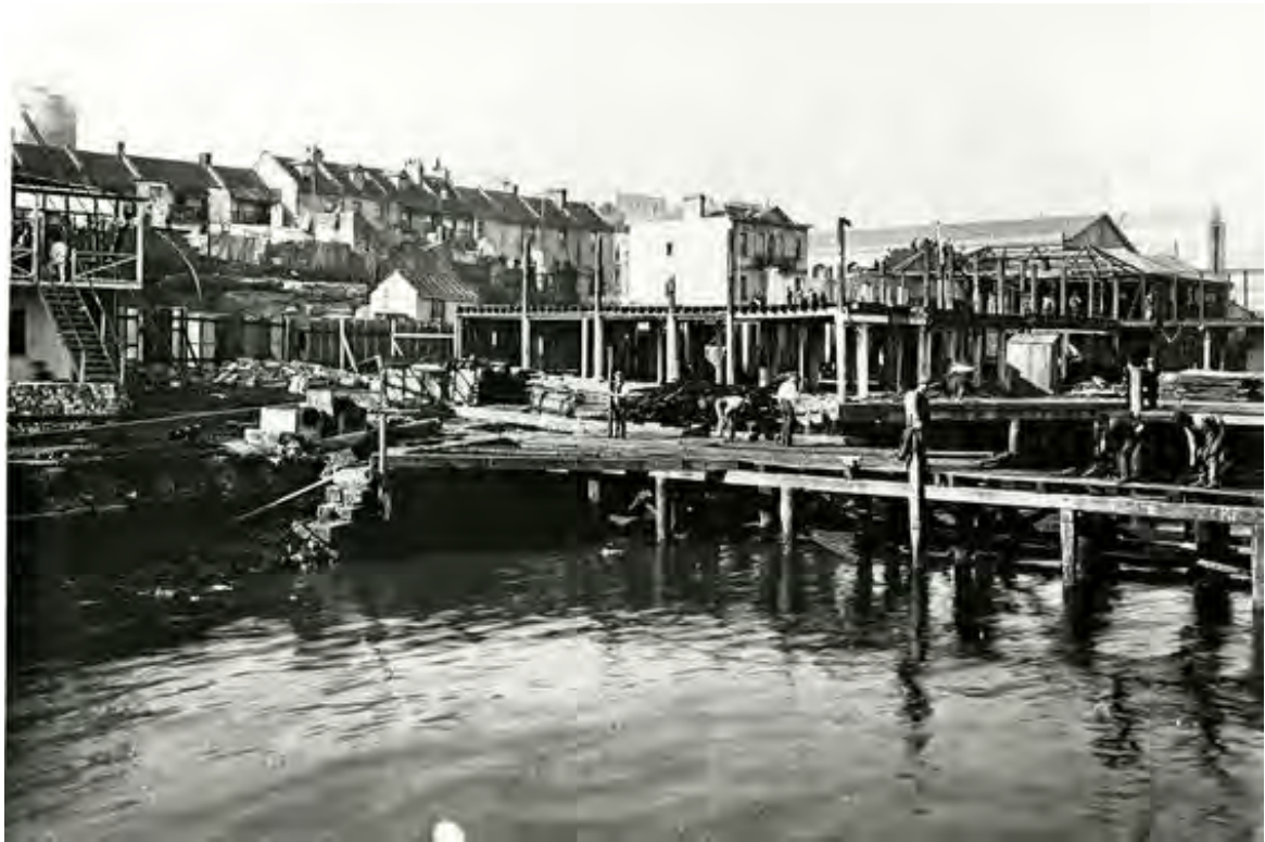
Figure 3.22. Demolition of the AS&N Co wharf 1910. The timbers on the wharfs and surrounding buildings are being lifted and taken away. Much of the timber was reused (Source: State Library of NSW GPO 1-48303)
