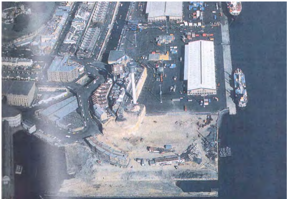
Figure 3.27. Excavation and reconstruction of the headland in the 1970s. Moore's Wharf has not been relocated and the surviving buildings are indicative of the former shape of the headland. (Source: Maritime Services Board Annual Report 1977-78, p 8)
