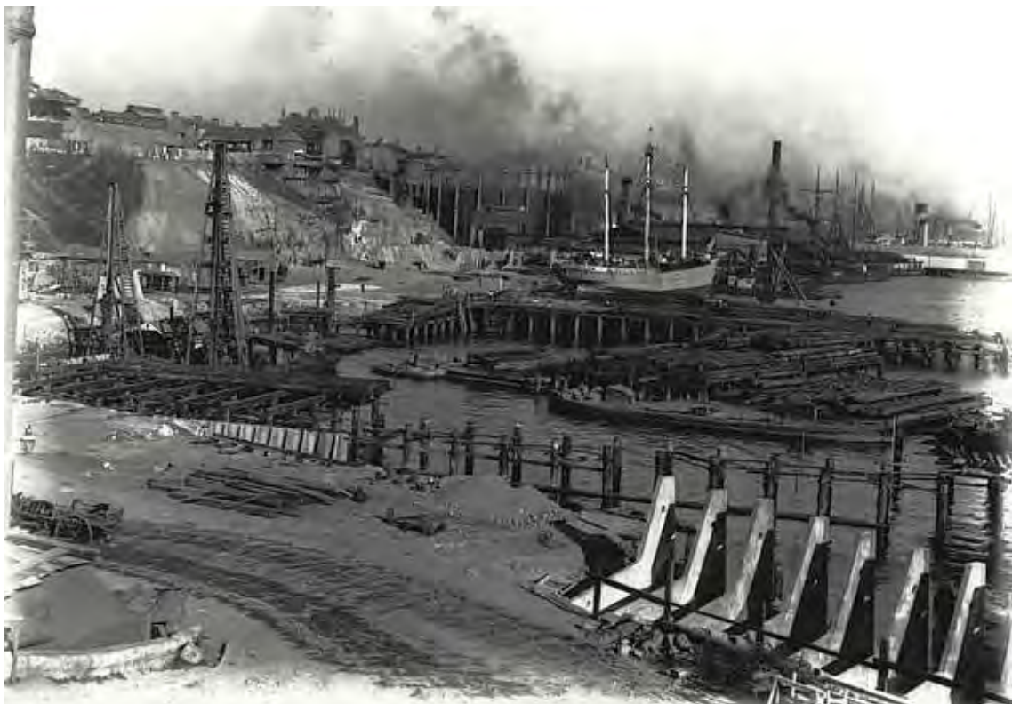
Figure 3.25. Construction of new wharfs at Darling Harbour c1912 with the gas holder and gas works in the background. Land has been reclaimed before the wharfs are constructed. Hickson Road is not yet formed and many of the old wharfs are still in place (Source: State Records ao17-AO17000007).
