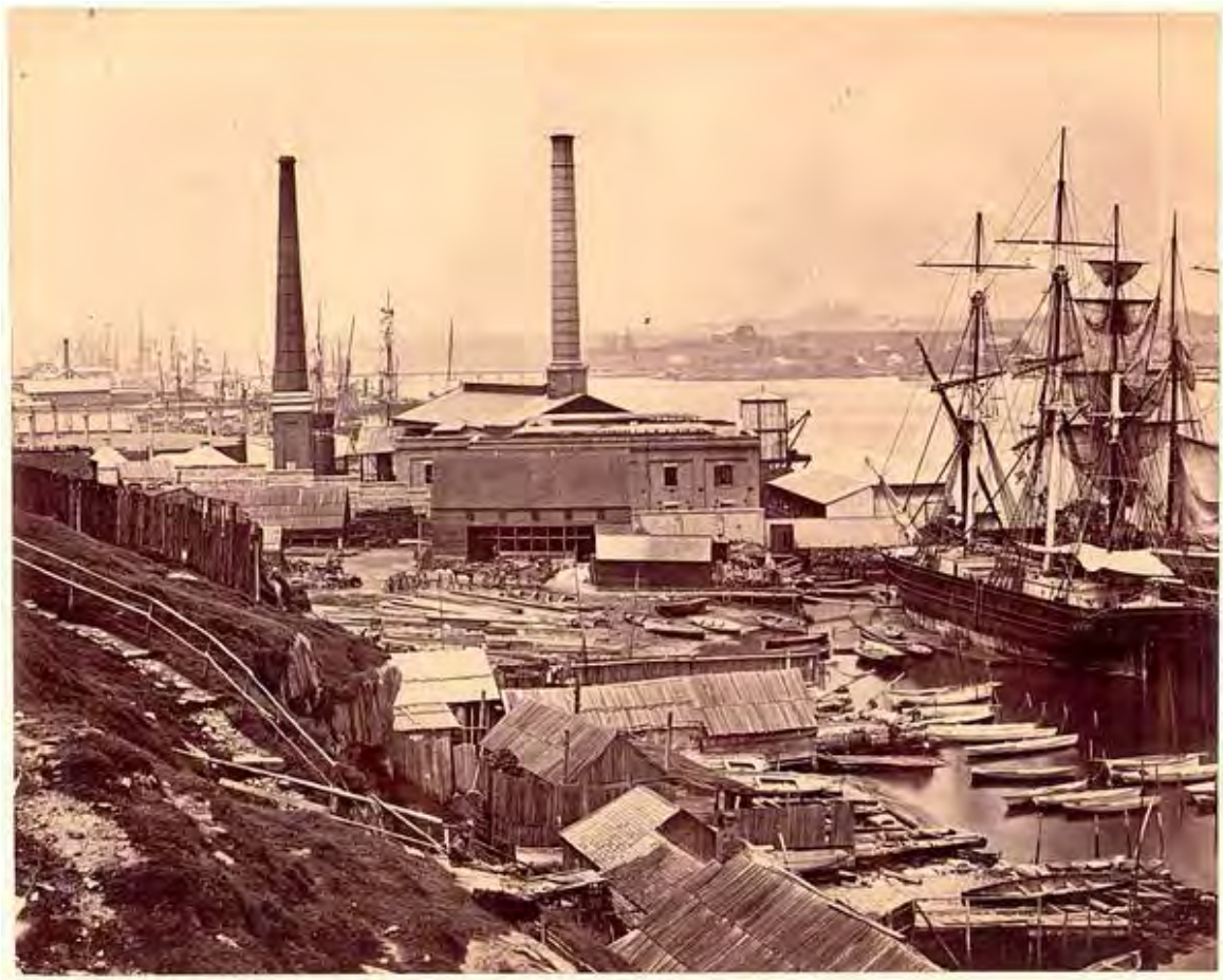
Figure 3.18. View to the south of the gas works around 1870. The large ships are moored at Rowntree's floating dock which was owned for a time by Cuthbert. The steep slope down to the harbour is traversed by stairs and a path with a handrail. Fencing appears to have been constructed around cliff edges. The gas works is constructed on reclaimed land (Source: State Library of NSW)
