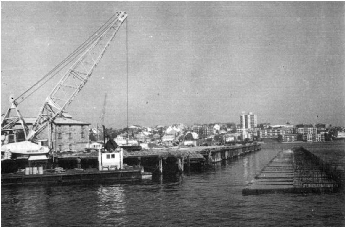
Figure 3.26. Repair of the northern edge of the wharf in the 1970s showing both timber and concrete piles (Source: State Library of NSW MP115).
