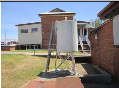
Photograph 11: Shows the 1,500L diesel AST.
