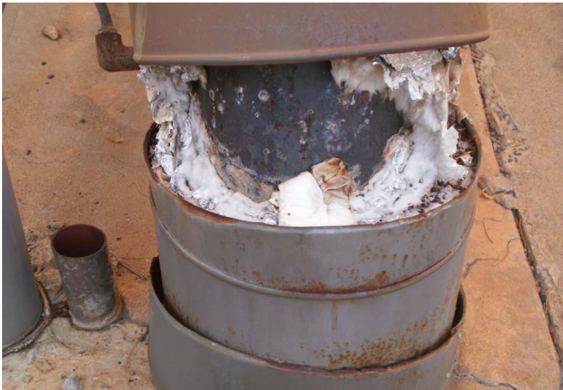
Photo 10/4 - Close up view of exposed insulation (assumed not to be ACM)
