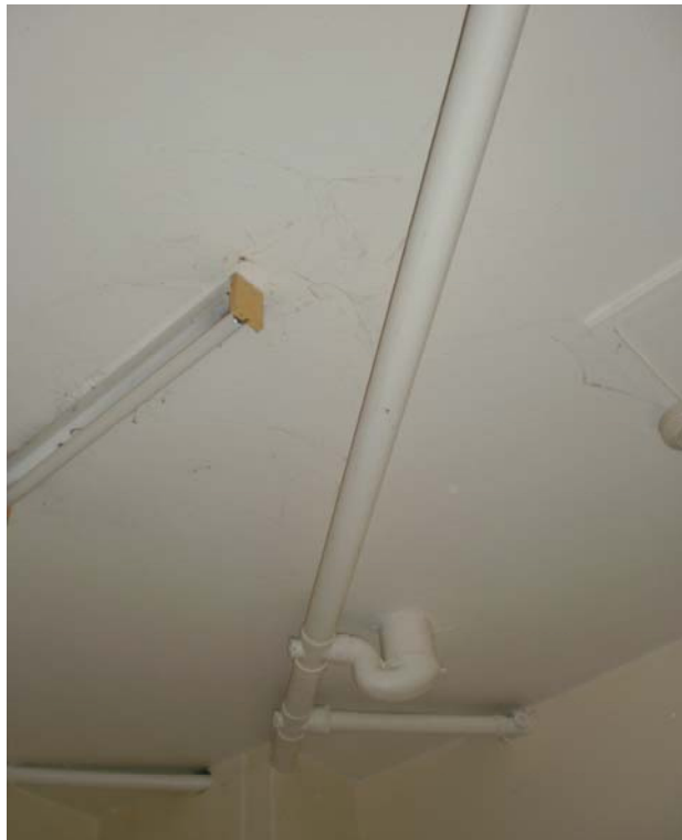
Photo 14/16 - Friable asbestos pipe lagging in bathroom
