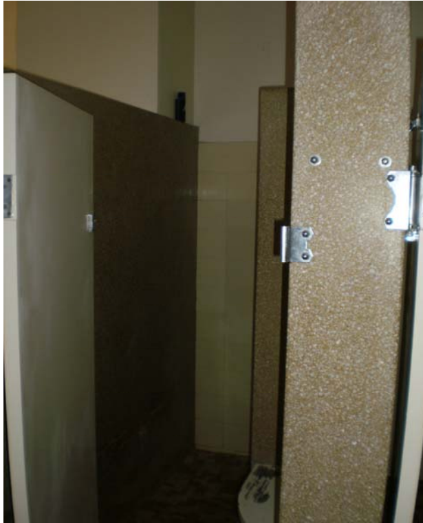
Photo 14/15 - Bonded asbestos partitions in bathroom
