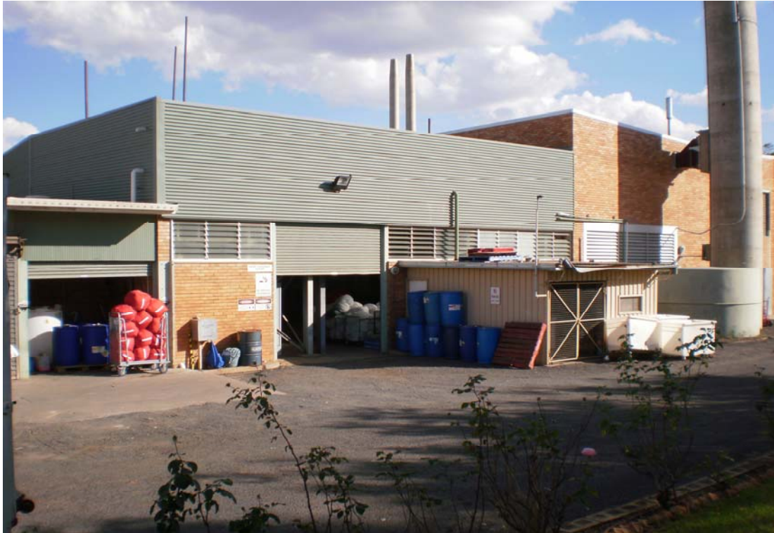
Photo 11/1 - Old boiler room adjacent to smoke stack (bonded asbestos pipes from building to stack)
