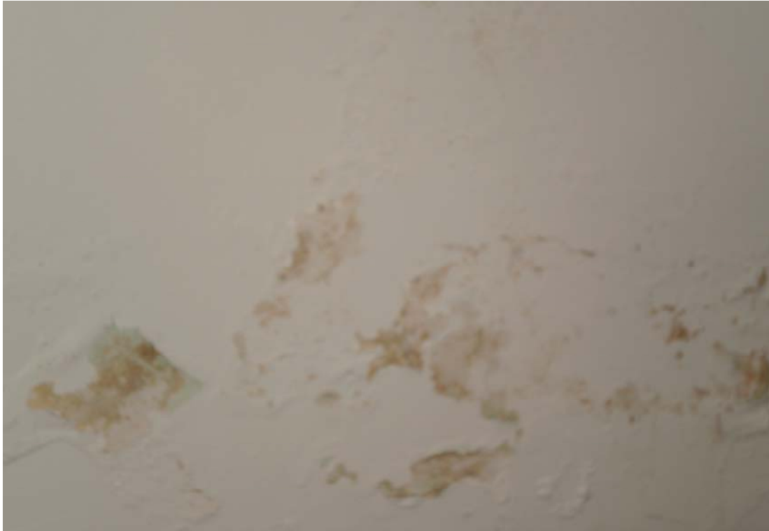
Photo 14/7 - Typical example of peeling paint (potentially lead-based)
