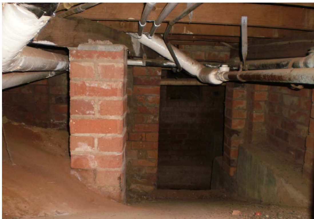
Photo 14/12 - Friable asbestos lagging in underfloor area
