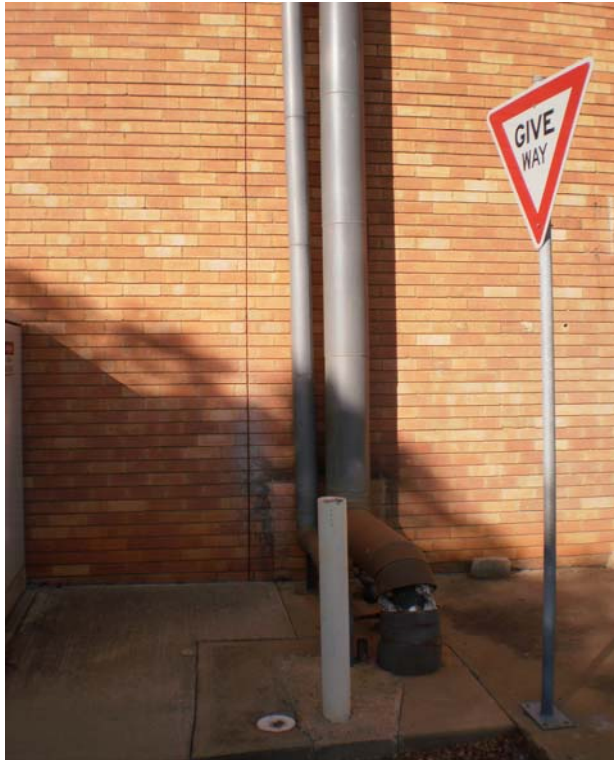
Photo 10/3 - Pipe with exposed insulation
