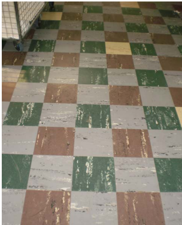
Photo 13/3 - Asbestos vinyl floor tiles
