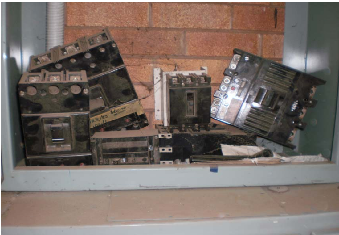
Photo 12/2 - Bakelite switches (potentially bonded asbestos + phenol)
