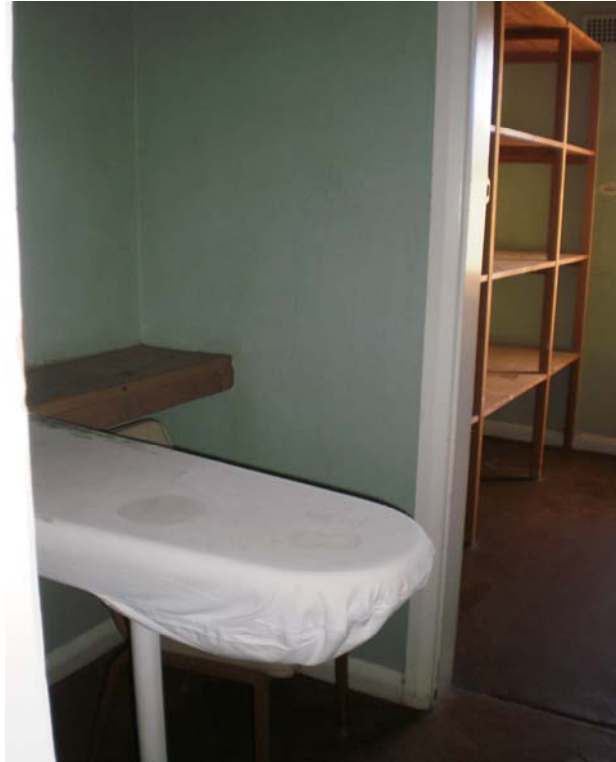
Photo 14/17 - Bonded asbestos partitions in laundry
