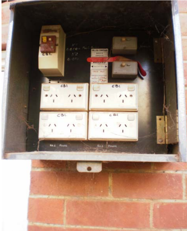
Photo 14/9 - Electrical switchboard (potentially bonded asbestos mounting board)
