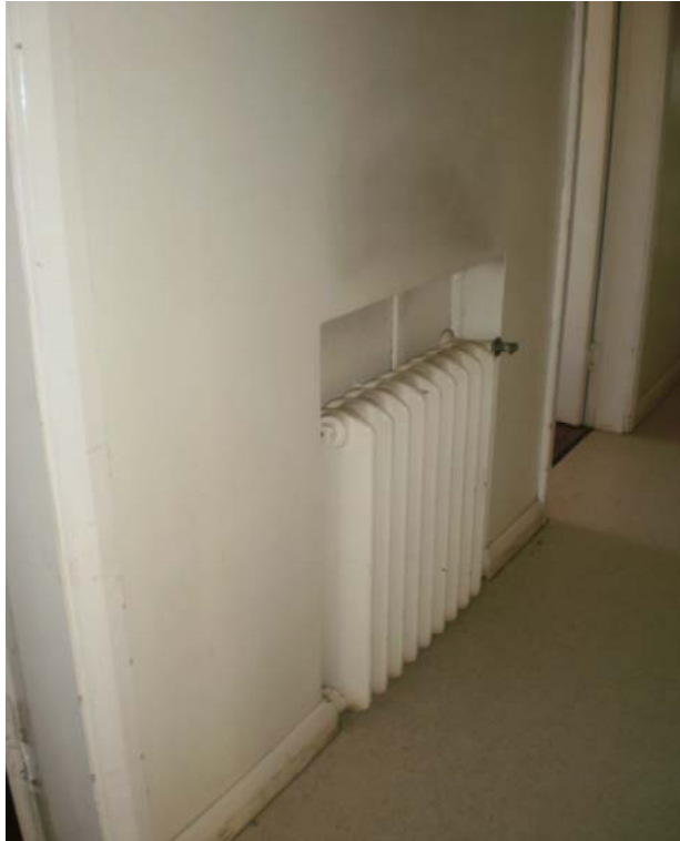
Photo 14/5 - Typical corridor heater (friable asbestos lagging on concealed pipes)
