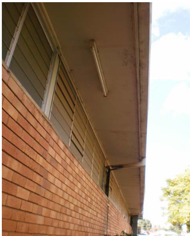
Photo 13/2 - Bonded asbestos eve lining
