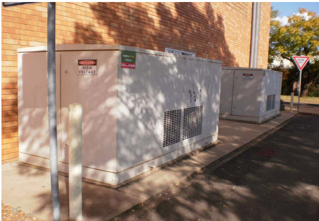
Photo 10/2 - Substations outside building
