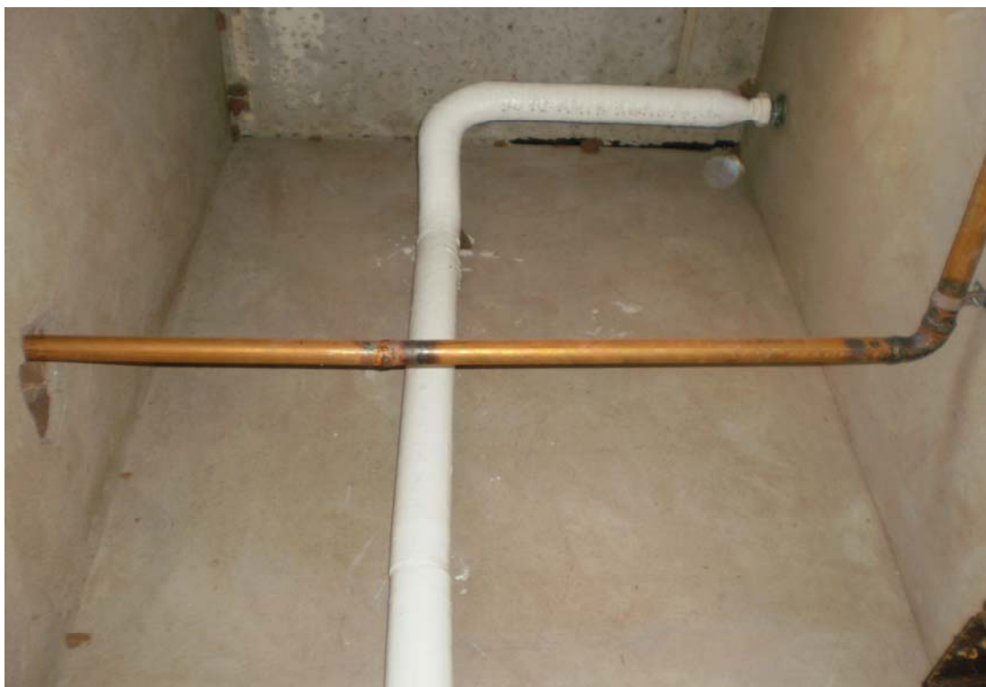
Photo 14/11 - Friable asbestos lagging in underfloor area
