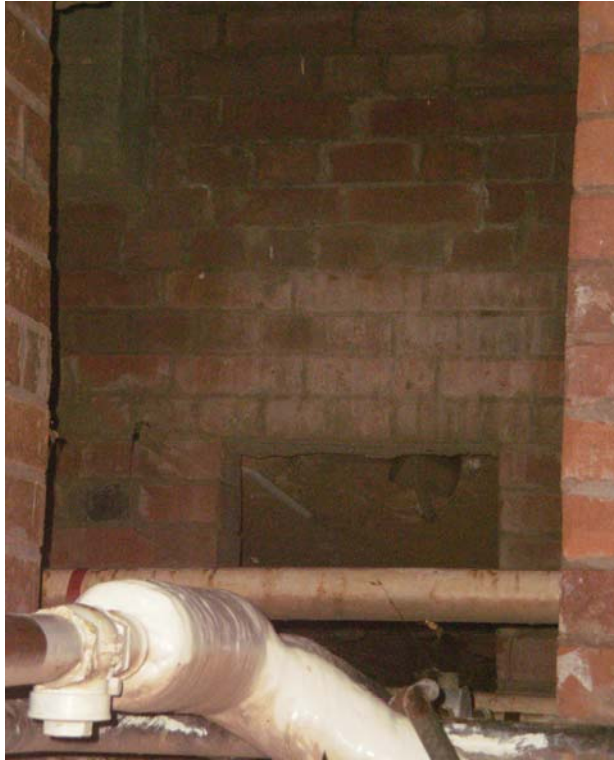
Photo 14/13 - Friable asbestos lagging in underfloor area (note lagging on ground)
