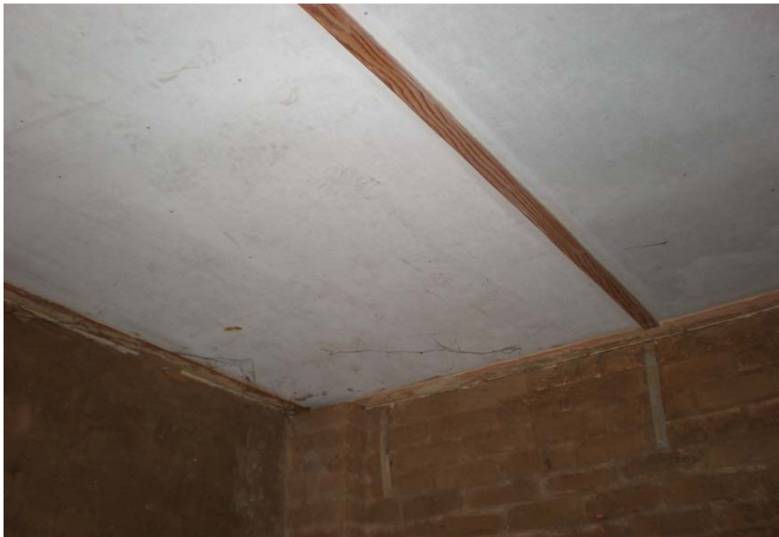
Photo 9/2 - Bonded asbestos ceiling inside electrician's store
