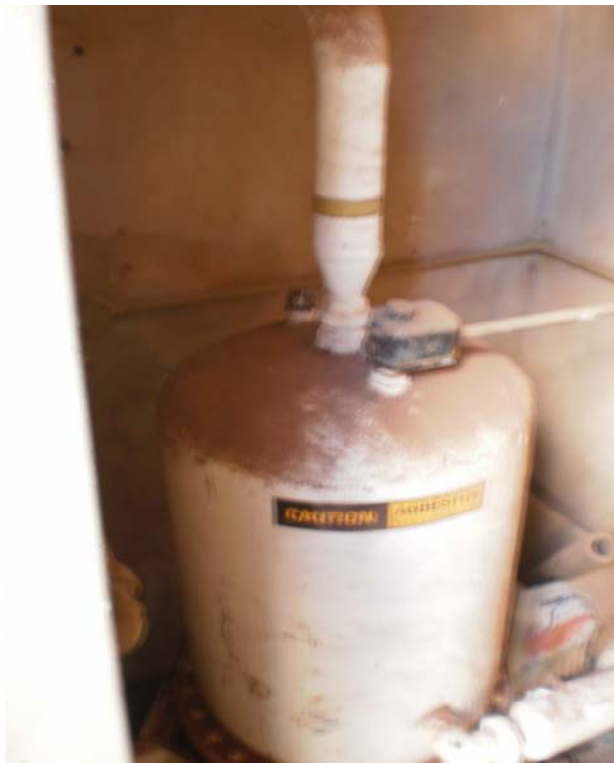
Photo 14/10 - Heat exchange unit (internal and external friable asbestos lagging)
