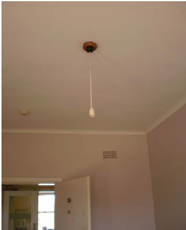
Photo 14/4 - Bakelite light fitting (potentially bonded asbestos + phenol)
