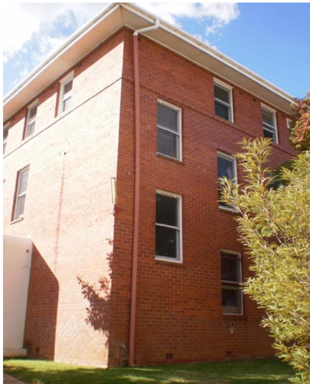
Photo 14/8 - View of bonded asbestos eave lining
