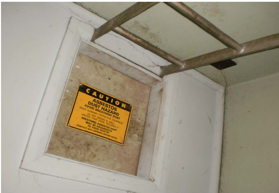
Photo 14/6 - Manhole to ceiling space (friable asbestos lagging on pipes in ceiling)
