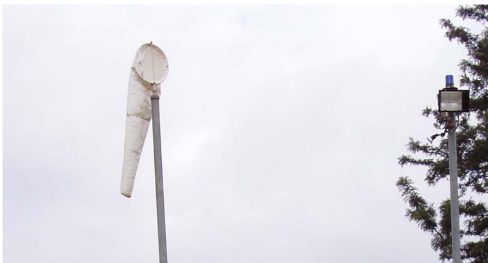
Figure 20: DBH HLS Windsock Lacking Necessary Illumination
