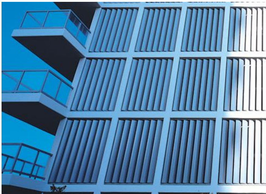
Figure 1 – Proposed aluminium louvres on the Tower 2 western façade Source: Candalepas Associates
