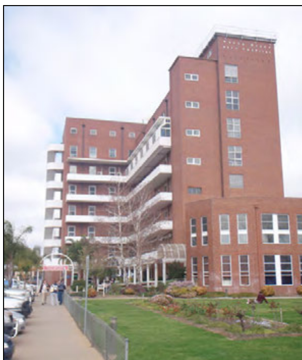
Figure 14: Looking south towards the Main Ward Building. The two storey section on the northern side, the fire stair and the ground floor colonnade are later additions to the original building.
