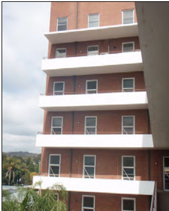
Figure 18: Detail of the eastern elevation, showing the regular pattern of triple hung windows and screen doors.
