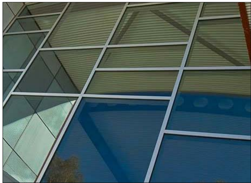
[GL1] GLAZING, WITH ALUMINIUM FRAMING PANELS: TRANSPARENT
