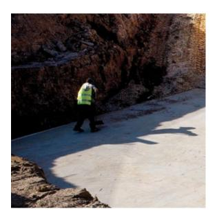
Lay a bead of StormMastic™ sealant on the slab approximately 60 mm inside the perimeter line marking.
