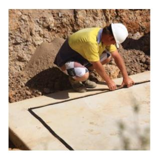
3. Secure the first module with four Swiftlift® anchors. Take care not to strike the modules together when you are unloading and lowering them. Be aware of pinch hazard at all times and don't walk or work under suspended loads.
