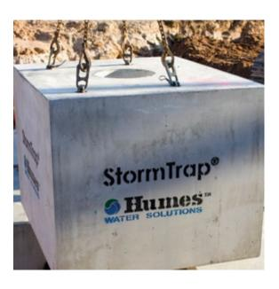
4. When lowering the first module into position, pause 50 mm above the concrete slab, then gradually lower it into position once it is aligned with the perimeter markings. Ensure the unit is square and the bottom of the module is on the foundation before you remove the lifters.
