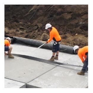
8. When four rows of modules have been laid, checked and sealed, backfilling can then occur (refer per note F. on page 2 of the approval drawings).
