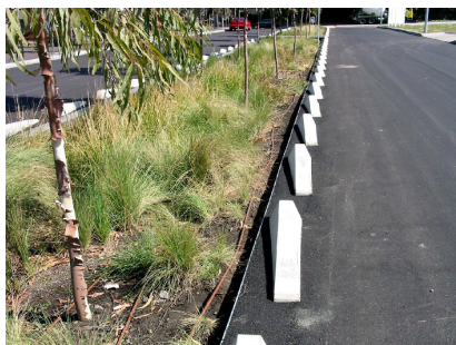
Figure 42: Water sensitive parking areas are required for parking layouts 100 cars of greater.
