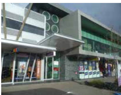
Figure 36: A break in the building form defines the pedestrian entry.
