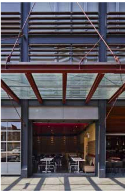
Figure 37: Exposed structural elements break down the bulk of a horizontal building form.
