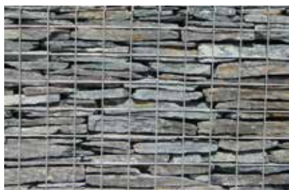
Figure 51: Low feature walls constructed of stone and other natural materials can contribute to the parklands character of the development.
