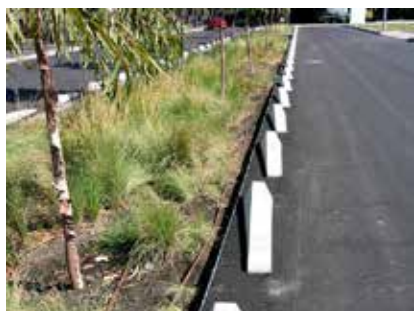
Figure 43: Water sensitive parking areas are required for parking layouts 100 cars of greater.
