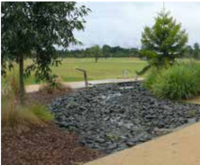
Figure 44: Ground materials can assist in the water run-off to planting areas.
