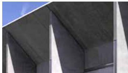
Figure 38: Exposed concrete is a durable material that can be used in a number of ways to articulate a building form.
