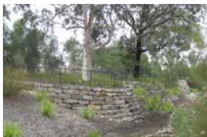
Figure 50: An example of fencing around a rock battered drainage channel.
