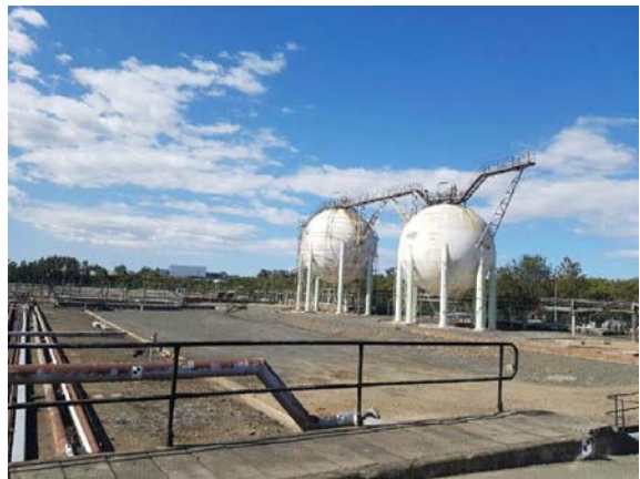
Figure 8 | View of the two LPG (butane) spheres (V137 and V140) (proposed to be demolished)
