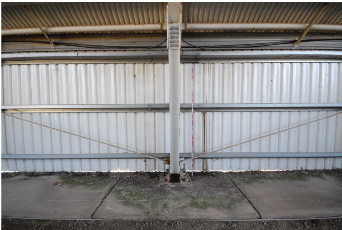
Figure 6.13 End-on view of column assembly, showing also cross bracing, (image no. STRARCH 0040)
