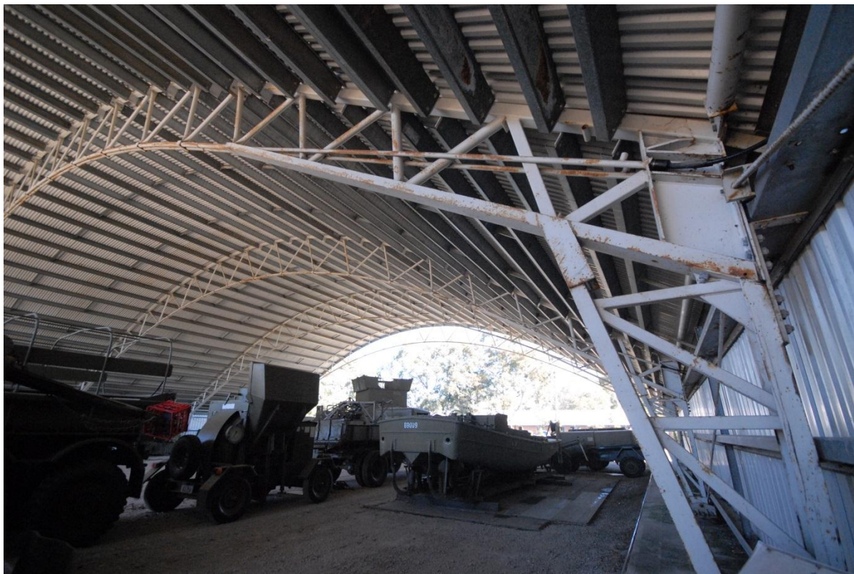
Figure 6.10 General interior view, looking SW, showing arch trusses, and columns, (image no. STRARCH 0028)
