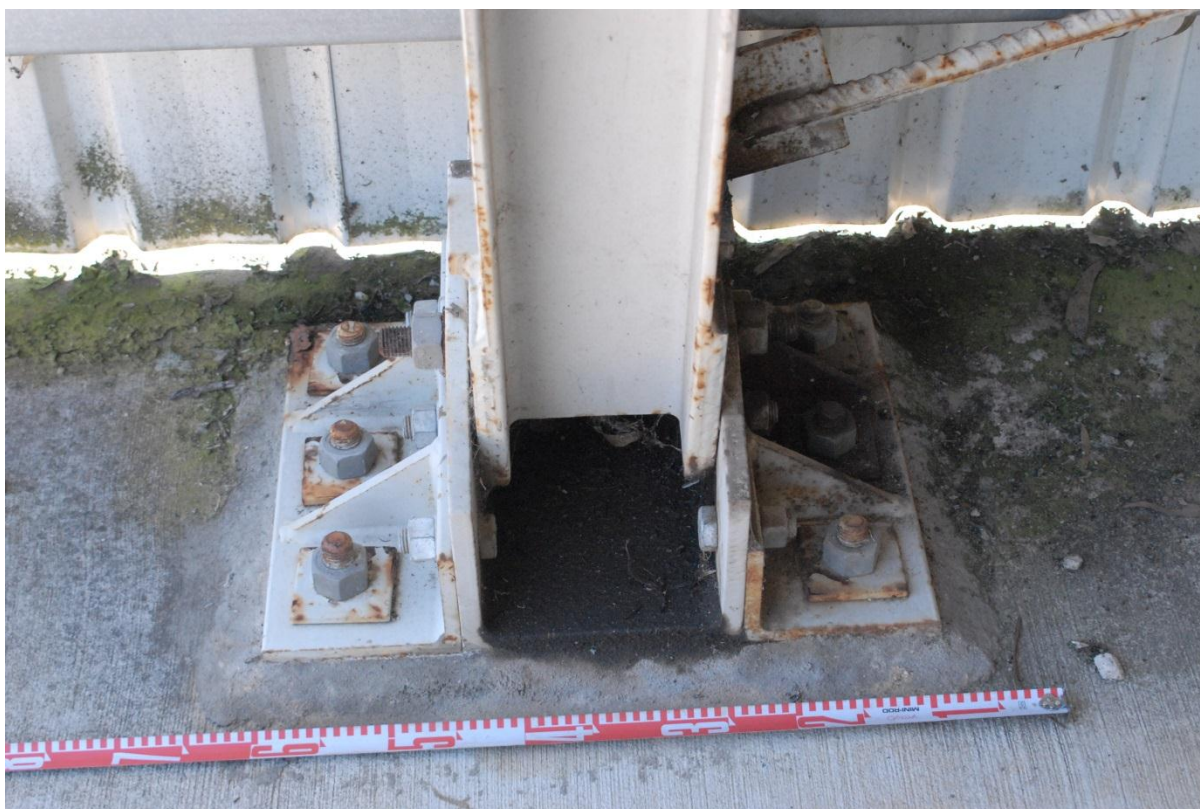
Figure 6.14 Detail of baseplate (image no. STRARCH 0046)
