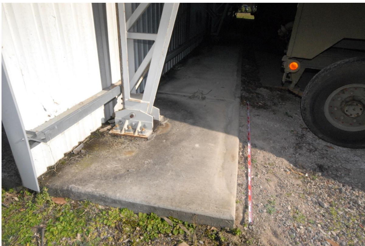
Figure 6.9 Detail view of SE corner of hangar showing lower column assembly, baseplate and concrete footing, (image no. STRARCH 0023)
