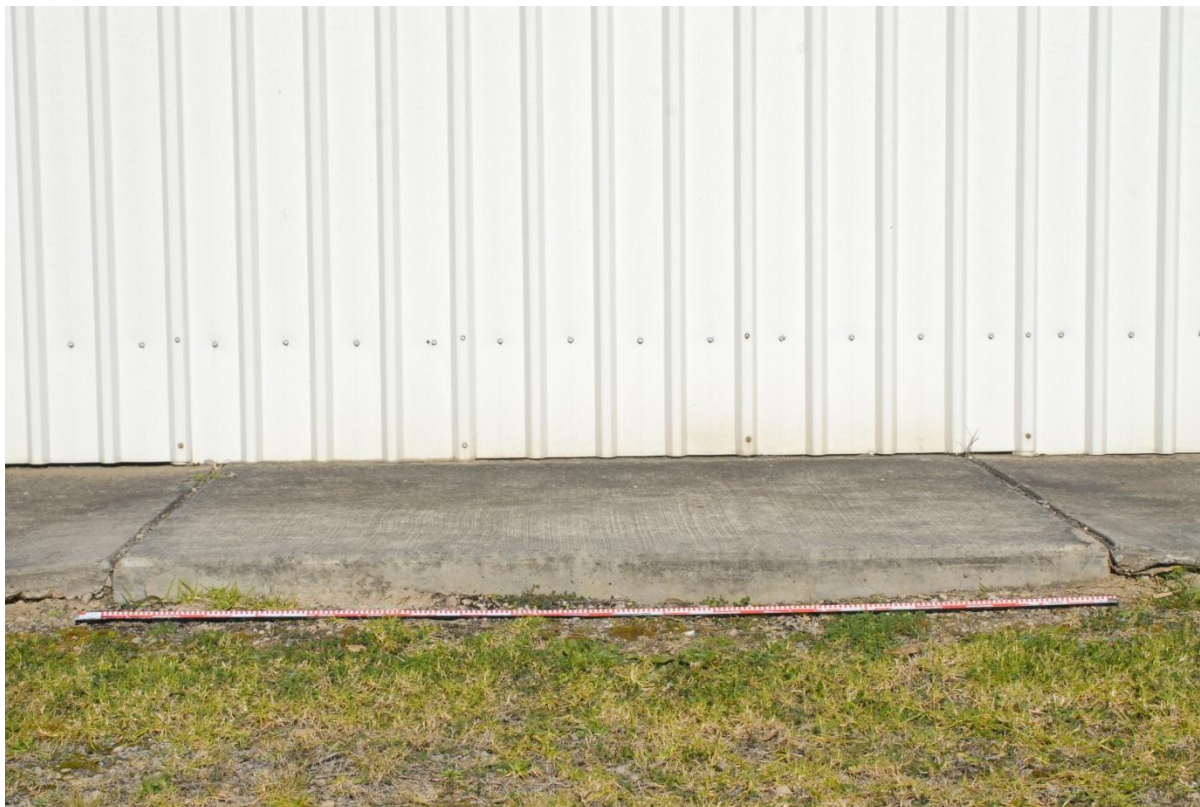
Figure 6.21 Exterior detail of a concrete footing with later paving 'infill' on either side, (image no. STRARCH 0073)
