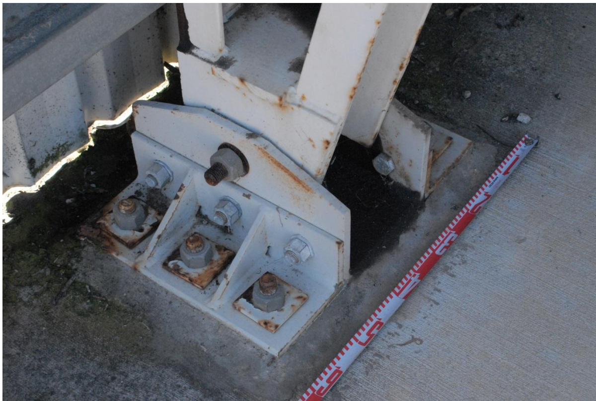
Figure 6.15 Side view of baseplate and horizontal pinning of column, (image no. STRARCH 0047)
