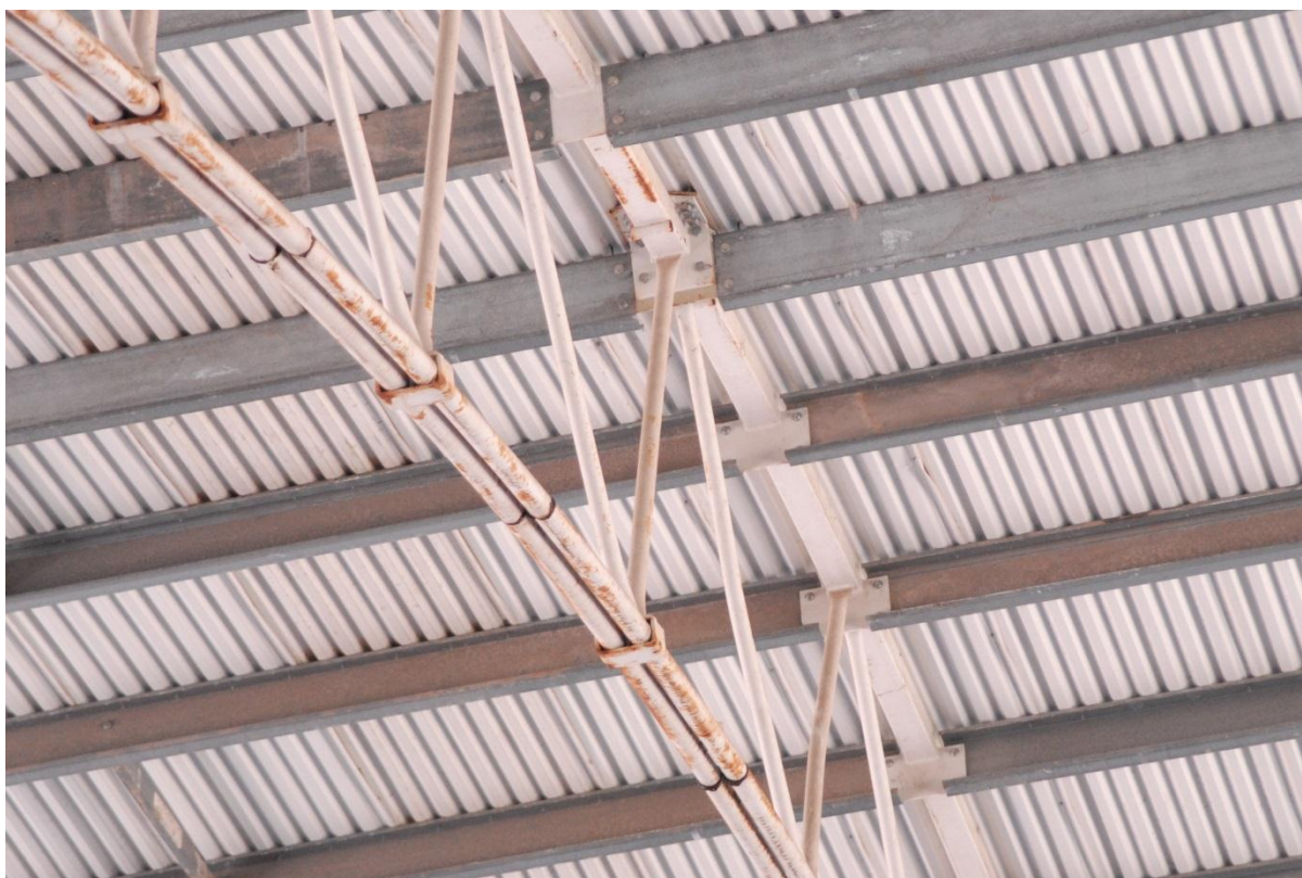
Figure 6.18 Detail of roof truss and purlins, (image no. STRARCH 0066)
