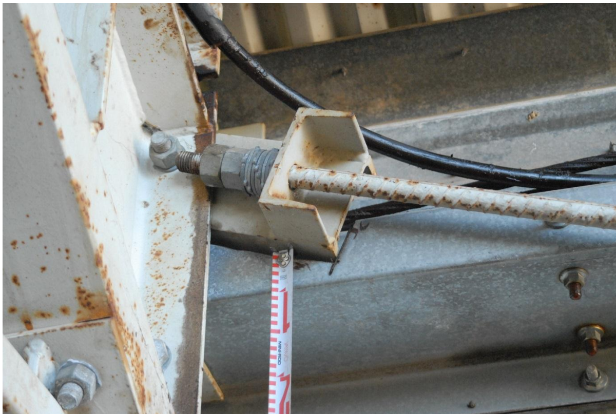
Figure 6.25 Detail of cross-bracing strut attachment to upper column assembly, (image no. STRARCH 0085)
