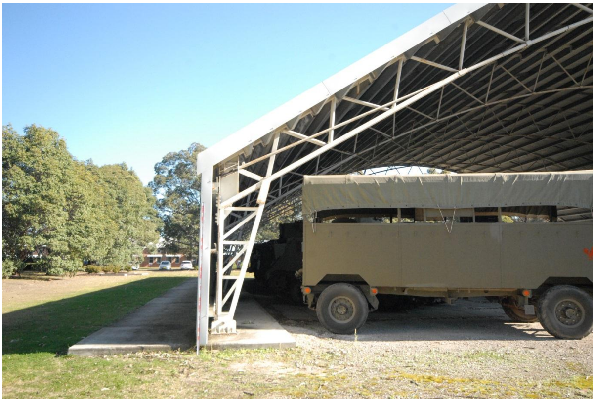
Figure 6.8 General side view of end trussed column assembly at SE corner of hangar, looking W, (image no. STRARCH 00019)
