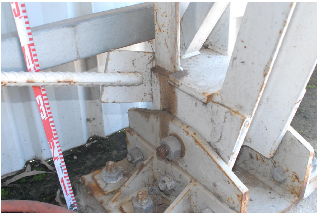
Figure 6.26 Detail of cross-bracing strut attachment to lower column assembly, (image no. STRARCH 0088)
