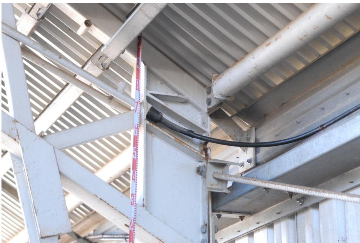
Figure 6.16 Detail of upper column, showing tensioning tendon and cross bracing strut, (image no. STRARCH 0060)
