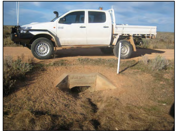
Figure 3.16: Example of Box Culvert
