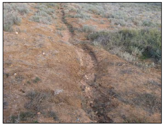
Figure 3.18: Example of Scour Downstream of a Culvert
