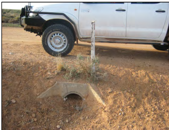
Figure 3.17: Example of Silted Culvert Inlet
