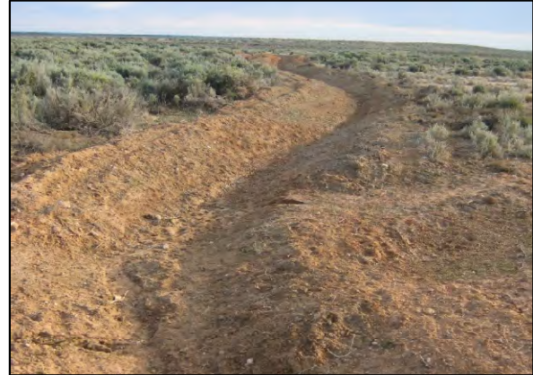
Figure 3.20: Example of Newly Constructed Outlet Drain
