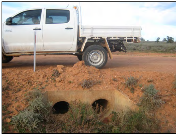
Figure 3.15: Example of Twin Circular Pipe Culvert
