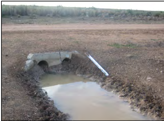
Figure 3.19: Ponding Downstream of a Culvert
