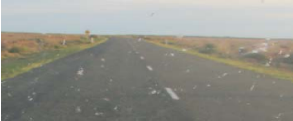
Photograph 6 Shadowing indicating some rutting in outer wheel path in sections
