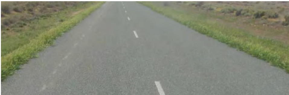
Photograph 2 Sections where vegetation in the shoulder restricts drainage
