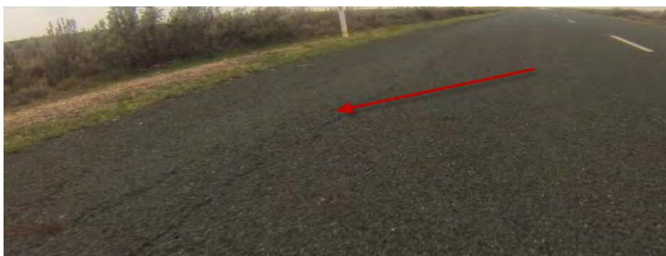
Photograph 5 Outer wheel path cracking
