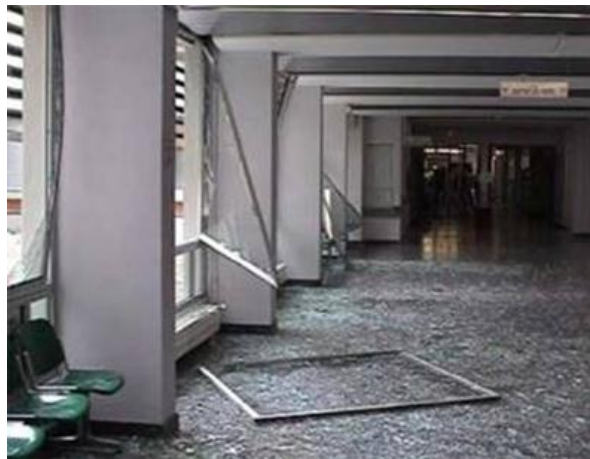
Figure 13: Damage from Flying Steel
