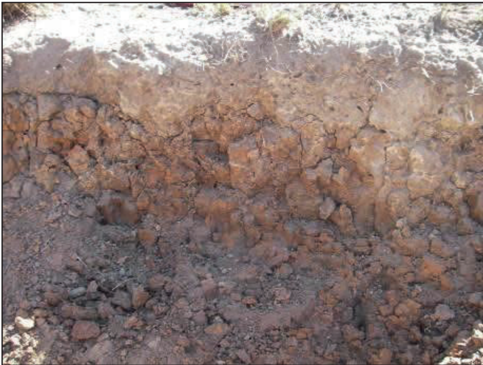
Plate 10: View into sectioned deposits (dam excavation) at the Buttonderry Site. Note the thin 'A' soil horizon (approximately 10cm), overlaying heavy clays.
