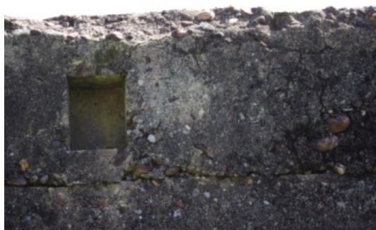
Image 4.37. Detail of pebble and shell aggregate with gap from former timber member. Facing northeast. Stedinger Associates, 2011 (File 2213).
