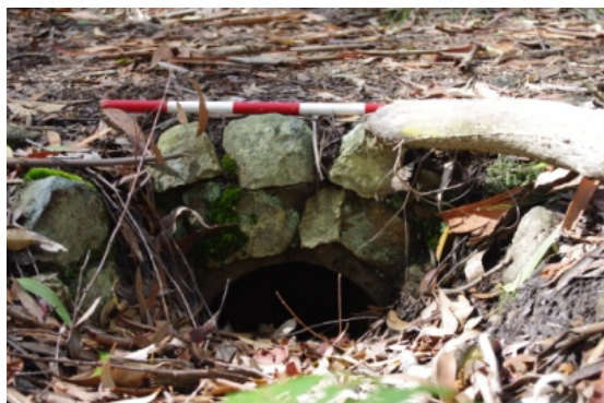
Image 4.29. A more recent culvert has been inserted along a track in Area 4. Facing south. Stedinger Associates, 2011 (File 2178).
