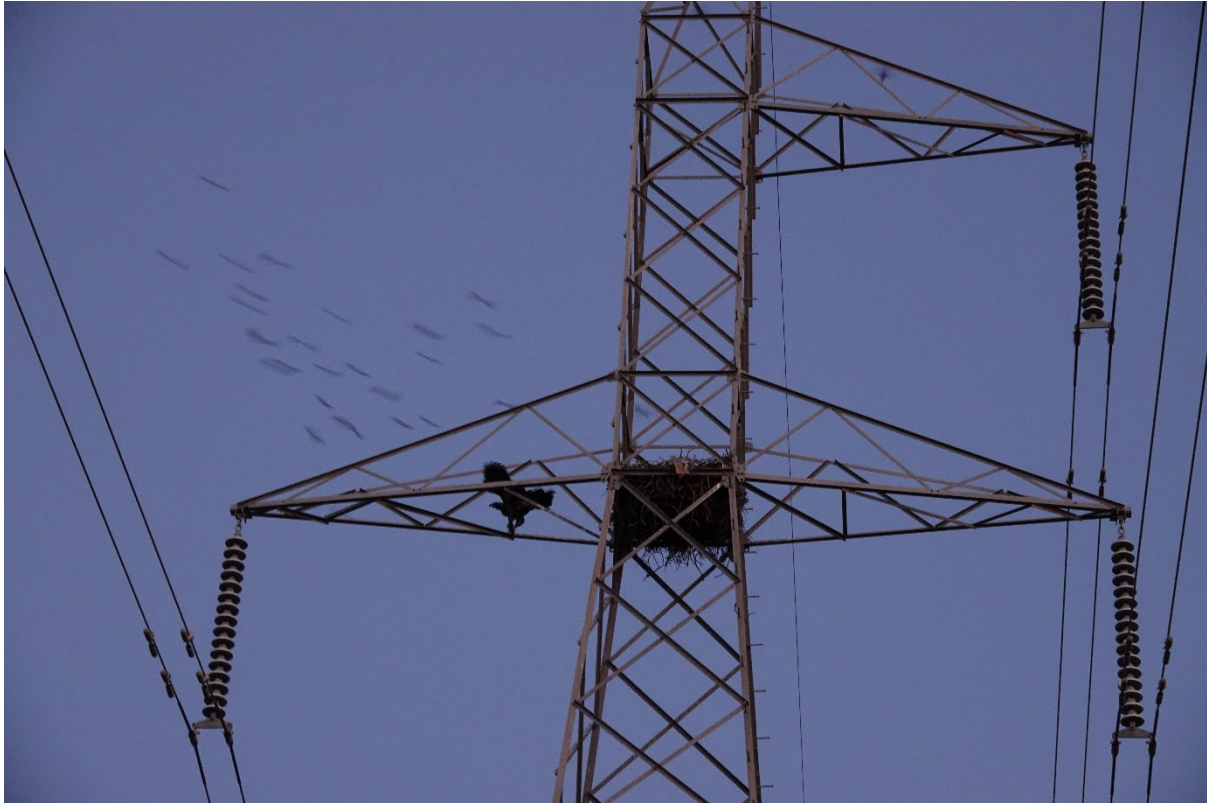
Photograph 4-3 Wedge-tailed Eagle Nest Observed during Spring 2021 Field Surveys on existing transmission tower.
