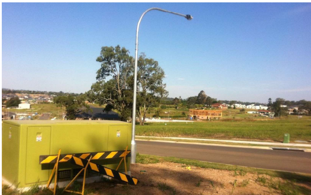
Padmount substations are converters of electricity, reducing the high voltages for street lighting and to the end user whilst low voltage pillar boxes are distribution junction points. These structures also mean underground cables are nearby. Digging activities and planting of trees or shrubs should not occur near them.
