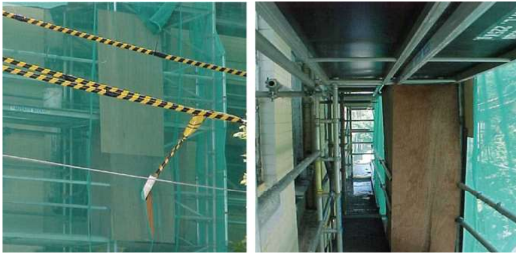
Figure 11 – Enclosure of overhead powerlines
