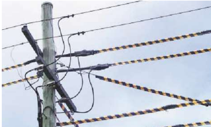
Figure 16 – Tiger tails fitted to overhead power lines
