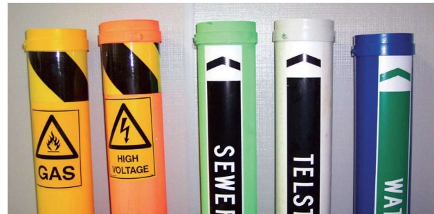
Colour Coded Conduits used to identify assets
