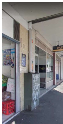
Example of 'awning' overhead power lines coming from a low voltage pillar on the road verge rising to through a duct and then through or above the awnings to the customer connection points for the premises. Source: Google Maps Street View.
