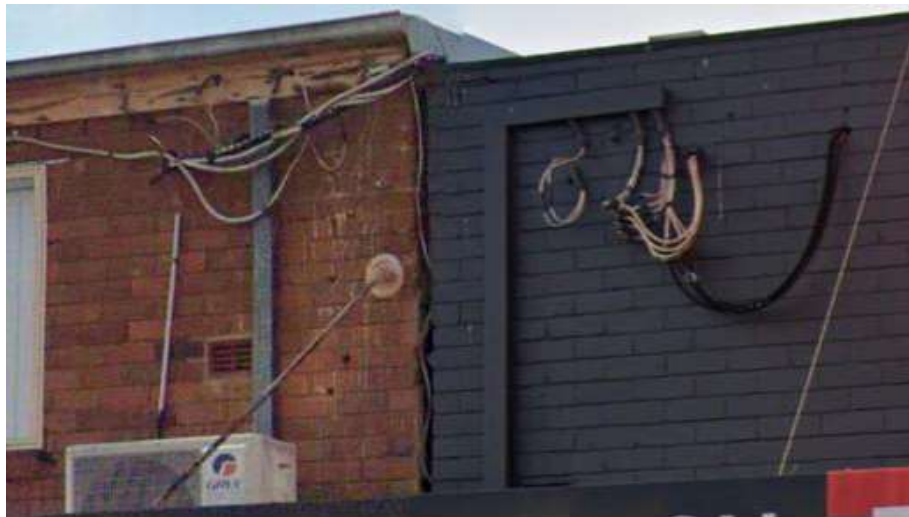
Example of 'awning' overhead power lines coming from a low voltage pillar on the road verge rising to through a duct and then through or above the awnings to the customer connection points for the premises. Source: Google Maps Street View.
