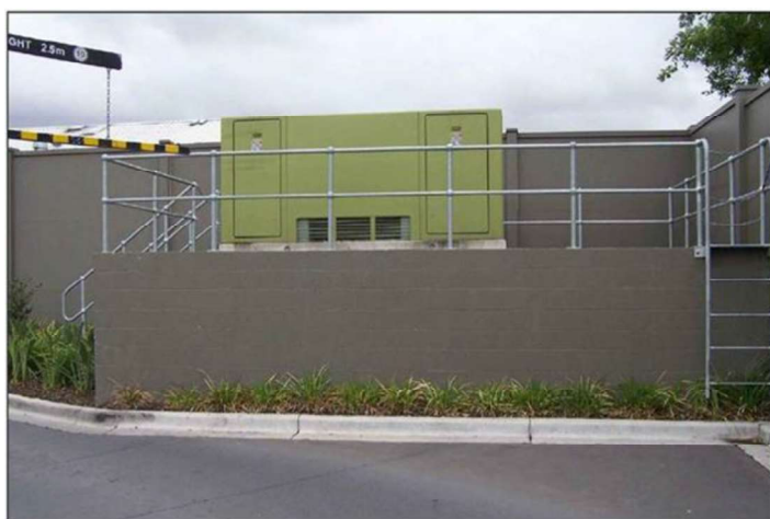
Figure 51 - Example substation raised above 1:100 flood level
