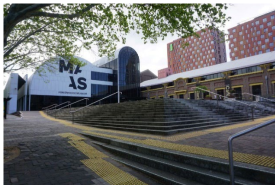
Figure 4.4: Existing surrounding built context of site, recent student housing multi-storey development visible behind Powerhouse buildings to east. View from Harris Street, Wran Building in back left. (Curio 2020)
