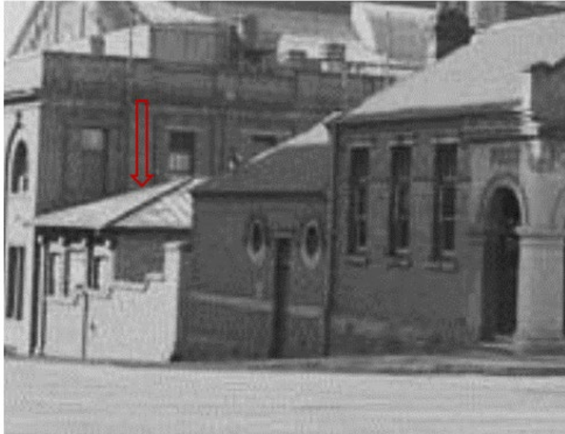
Figure 3.18: Tramway Induction Room between Office and Ultimo Post Office in 1947 (Source: NLA)
