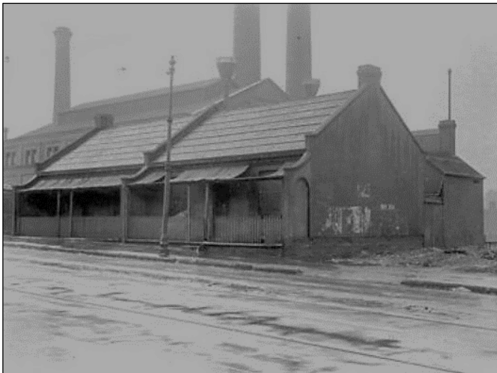
Figure 3.13: Semi-detached brick house pair at 554-556 Harris Street prior to demolition in 1922, with Ultimo Power House (Source: City of Sydney Archives NSCA CRS 51/992).
