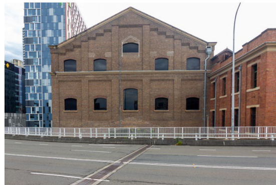
Figure 4.2 : Southern view of the Boiler House and North Annex from Pier Street (Curio 2020)
