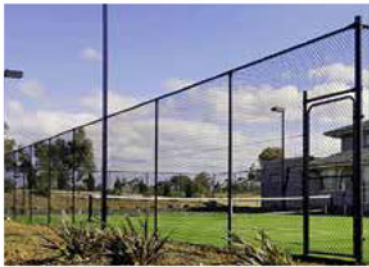
FENCE TYPE 3 2.4m high chainwire fence
