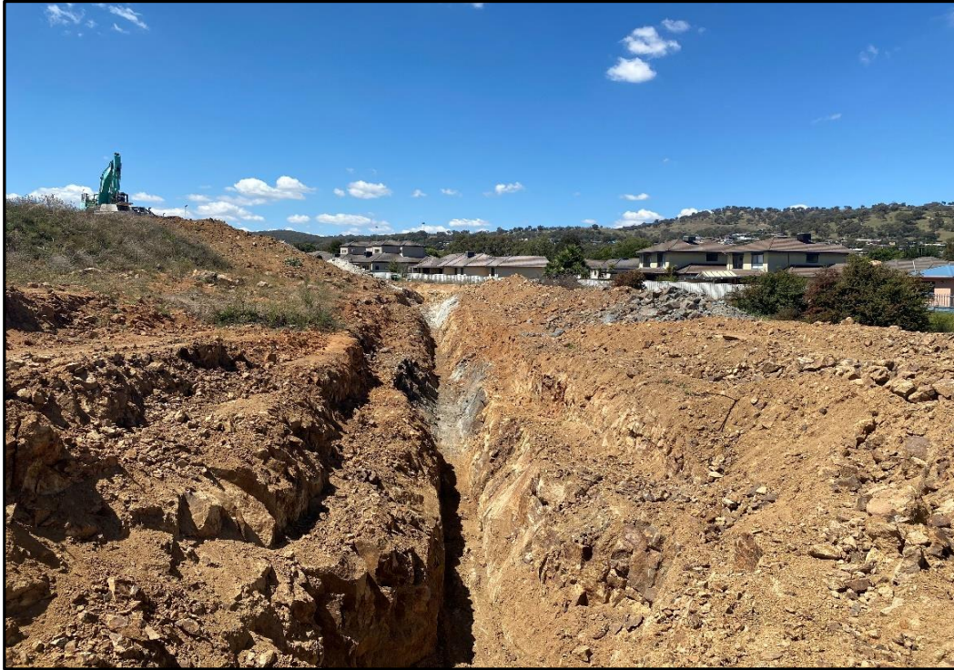
Photo 7: View of the trench excavation exposing residual soils and weathered rock
