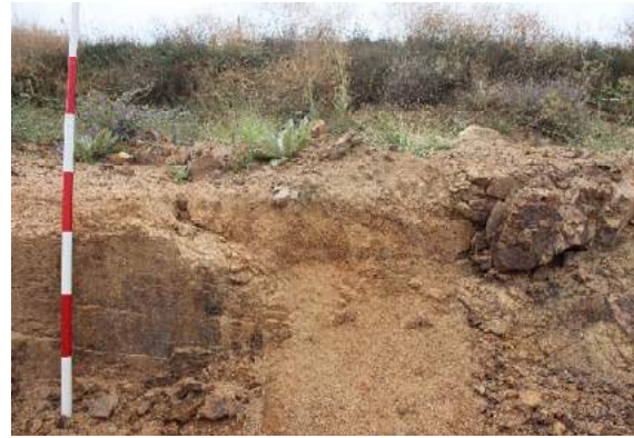
Figure 13: Exposure along the southern boundary of the study area along the excavated access track. Thin A horizon over clay loams and exposed bedrock.
