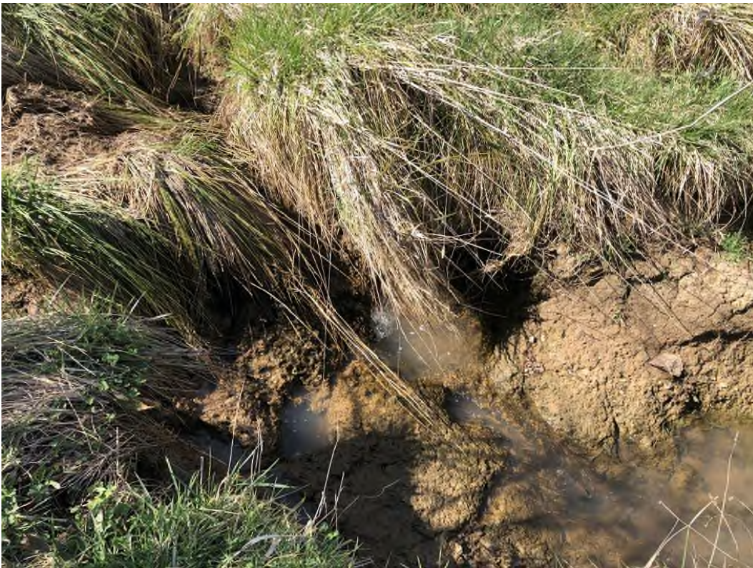
Figure 8: Eroded banks of the channel through the sedgeland
