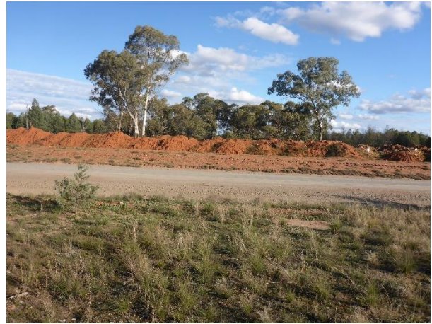
Figure 6-12: View south across SU2 showing heavy vehicle access road and topsoil stockpile
