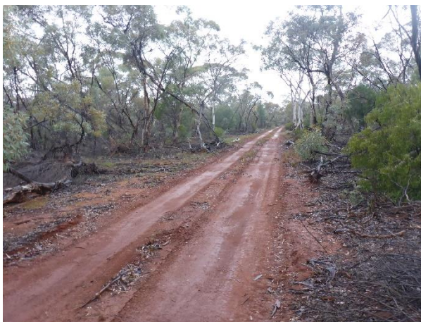
Figure 6-22: Existing access track into the Federation Site
