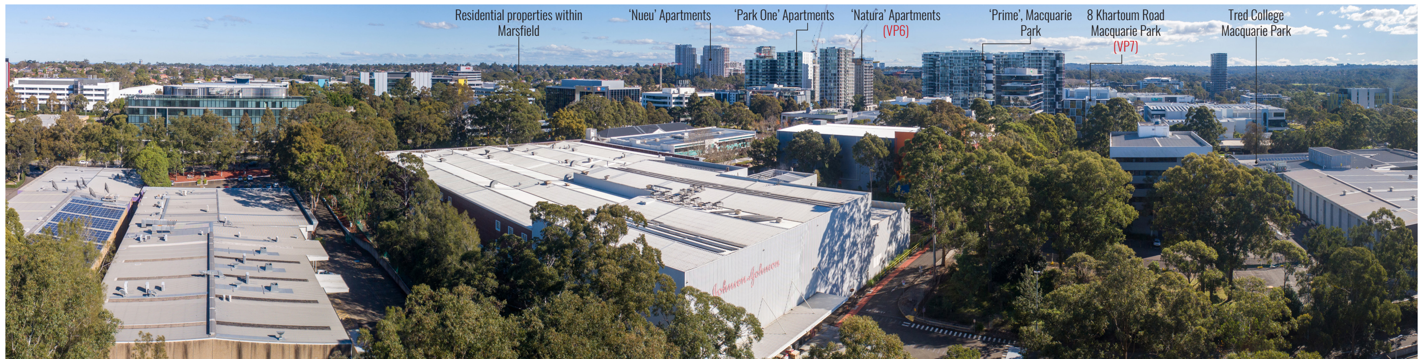
Figure 6: Drone at Position 1 - 45m AGL - Looking West
