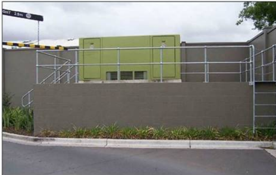
Figure 51 - Example substation raised above 1:100 flood level
