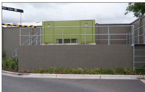
Figure 51 - Example substation raised above 1:100 flood level
