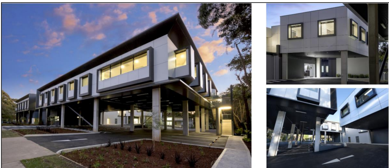
Figure 35 Photos of existing entry (Erilyan 2021)
