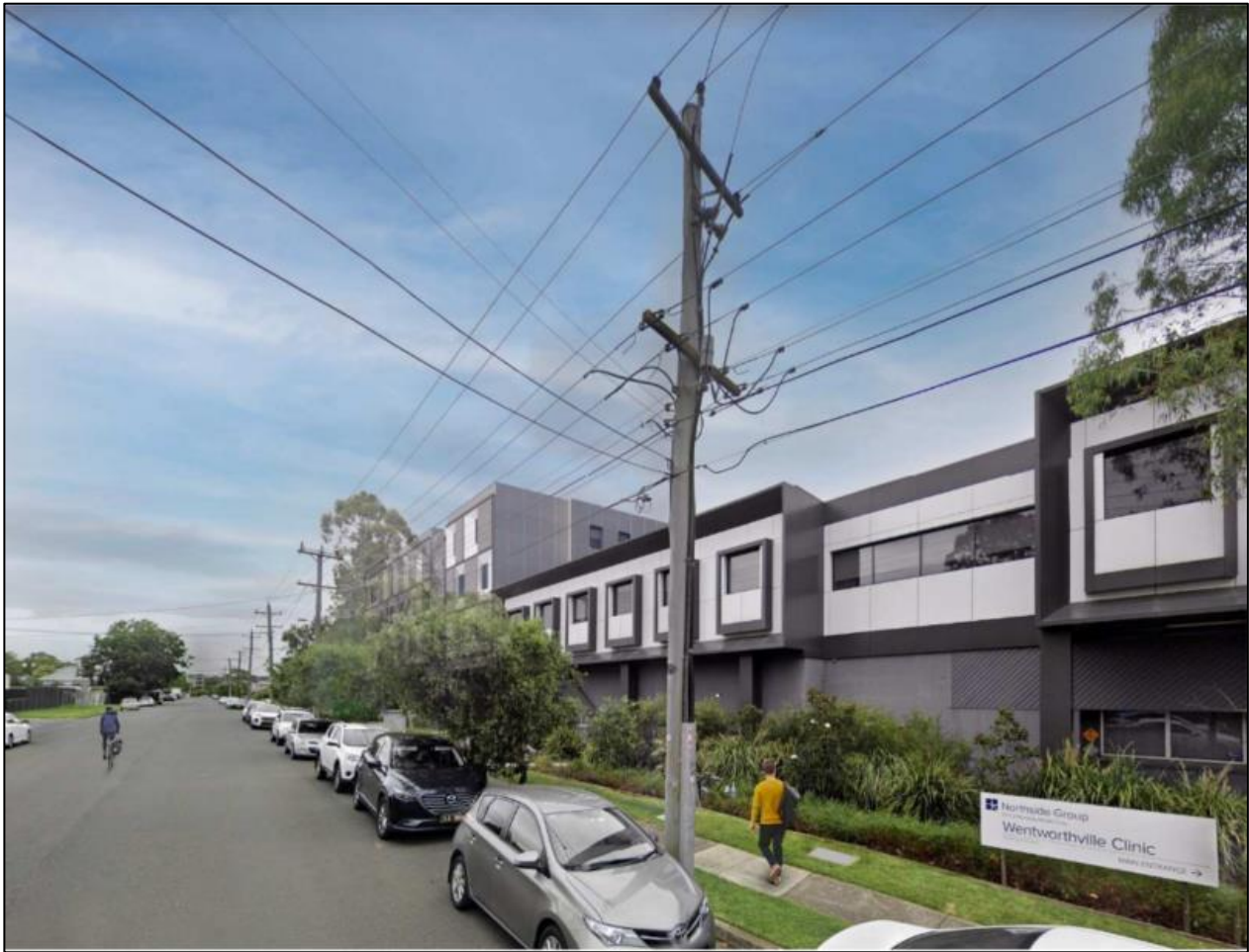
Figure 10 View from north east showing relationship with Stage 1 and Lytton Street (Team 2 Architects 2021)
