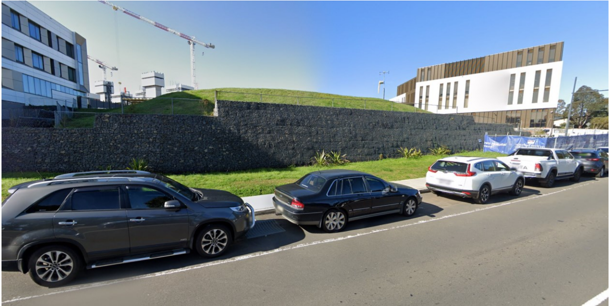
Figure 2: Looking west from Parkside Crescent (helipad is above gabion retaining wall and batter)
