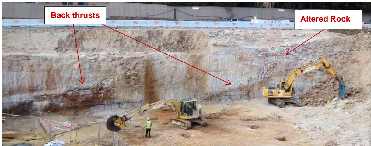
Figure 2: Back thrusts in an excavation wall at a nearby site
