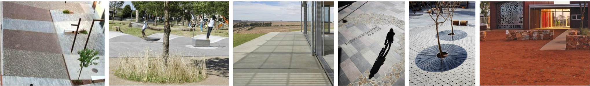
Combination of paving materials along promenade. Tree detail in hardscape. Seamless transition from inside blocks to external surfaces. Educational paving features. Porous paving around tree pits. Earthy coloured gravels and decomposed granite.
