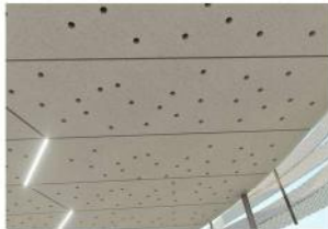
PERFORATED FC SOFFIT, FACTORY PAINTED
