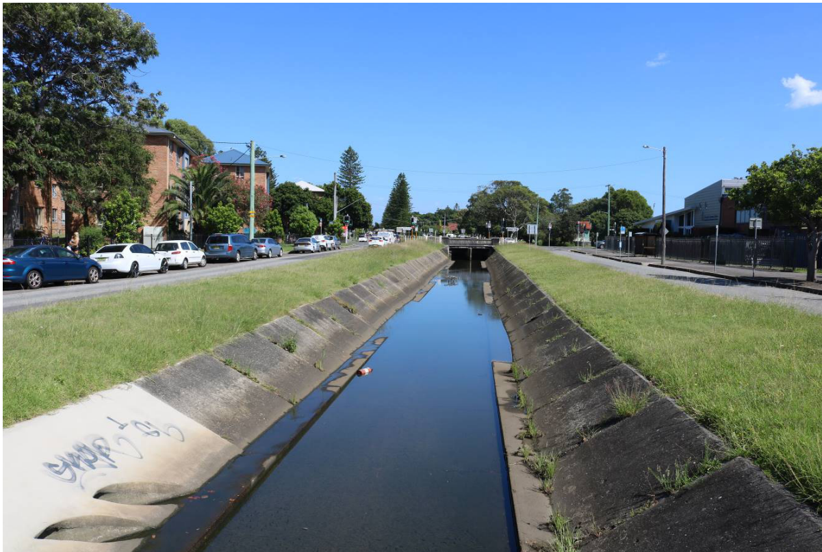
Photograph 4 – Parkway Avenue along site frontage.
