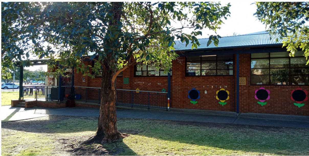
Plate 3 Single-storey brick building in central portion of Project Area
