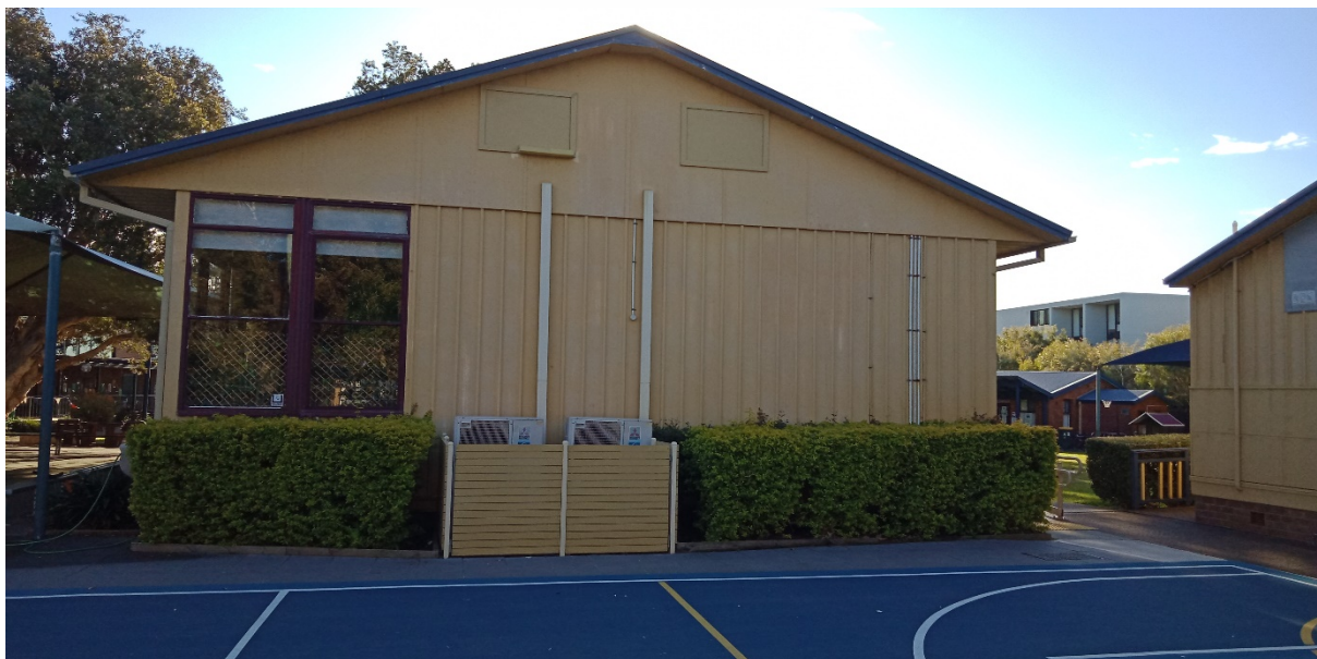
Plate 4 Sports court and classroom in south-eastern portion of the Project Area, view to north-west
