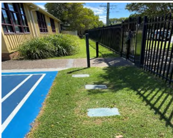
Photograph 1: View north east - Surface conditions along the eastern perimeter boundary
