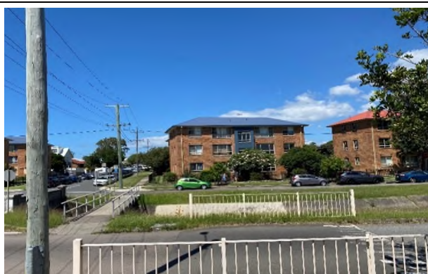
Photograph 4: View south east - Medium density residential dwellings and concrete stormwater drain Cottage Creek
