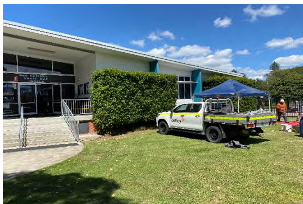
Photograph 8: View south west - Concrete and playground surface conditions. Main auditorium building in background
