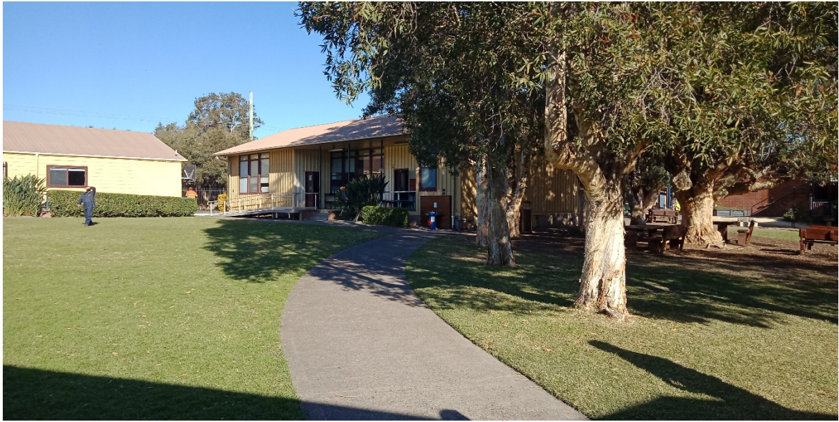
Plate 3 Single storey buildings at rear
