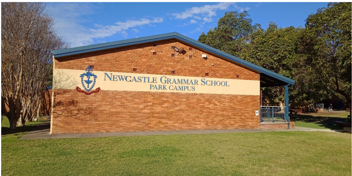
Plate 2 Single storey building at rear
