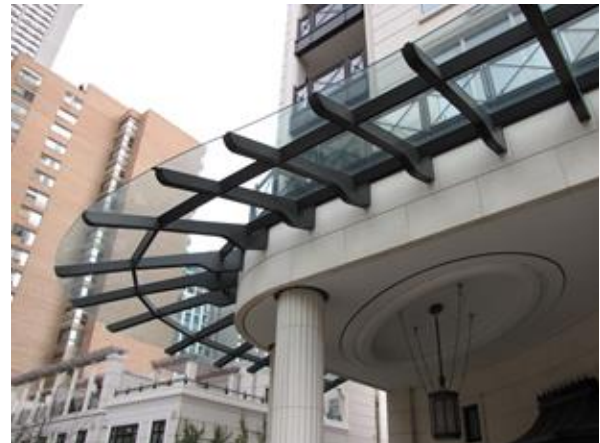
Figure 7: Examples of Corner Canopy and Wind Control Features at Building Entrances
