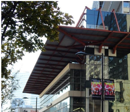
Figure 7: Examples of Corner Canopy and Wind Control Features at Building Entrances
