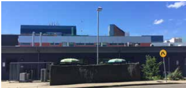
Fig 26: View of loading area
