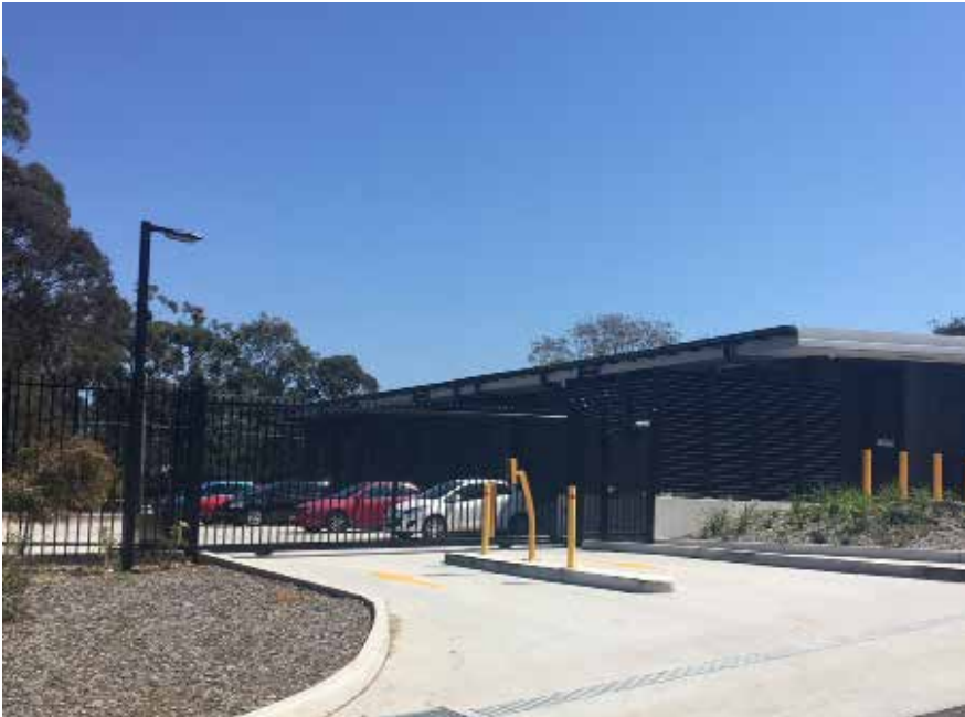
Fig 29: View of ambulance station
