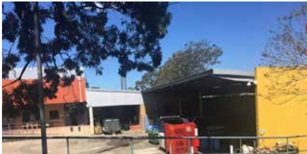
Fig 32: View of loading bay
