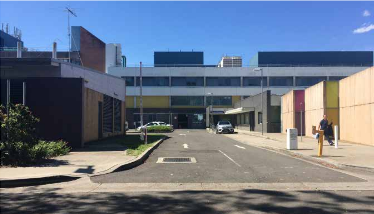
Fig 25: View of southern entry
