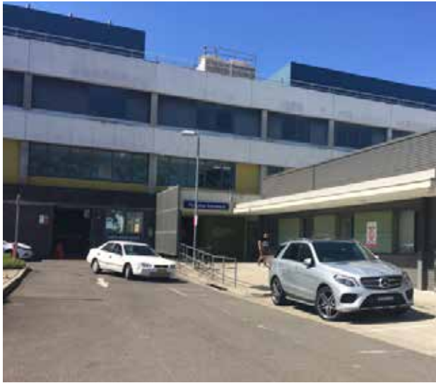
Fig 24: View of southern entry
