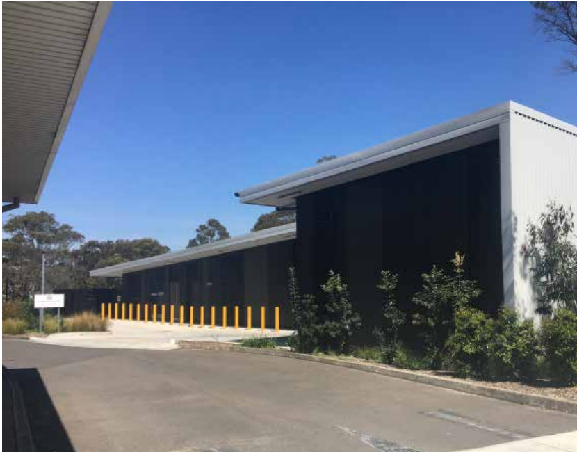
Fig 28: View of ambulance station
