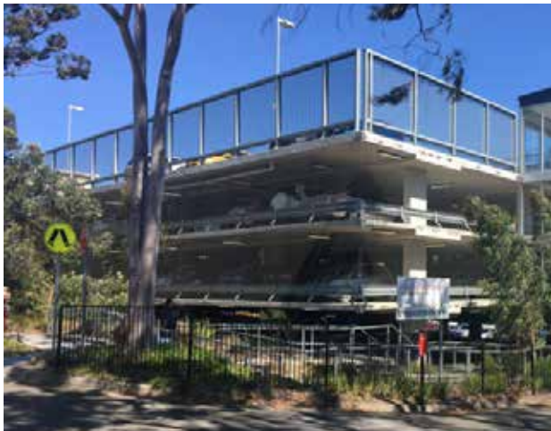
Fig 31: View of multi deck car park
