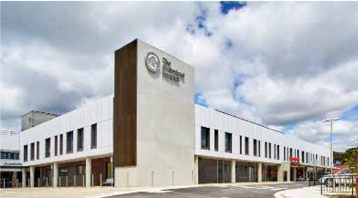
Fig 34: View of stage 1 building
