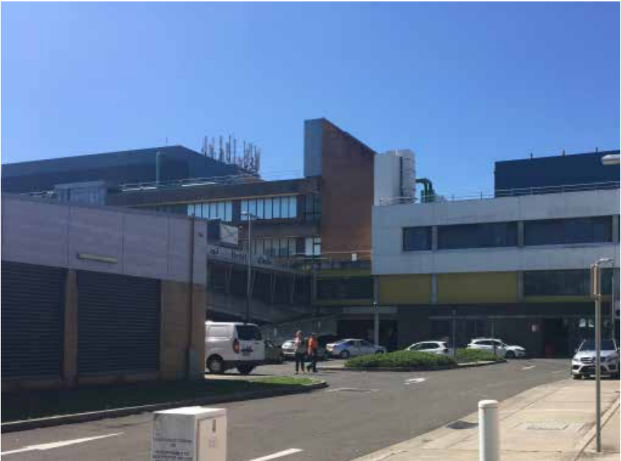
Fig 23: View of southern entry
