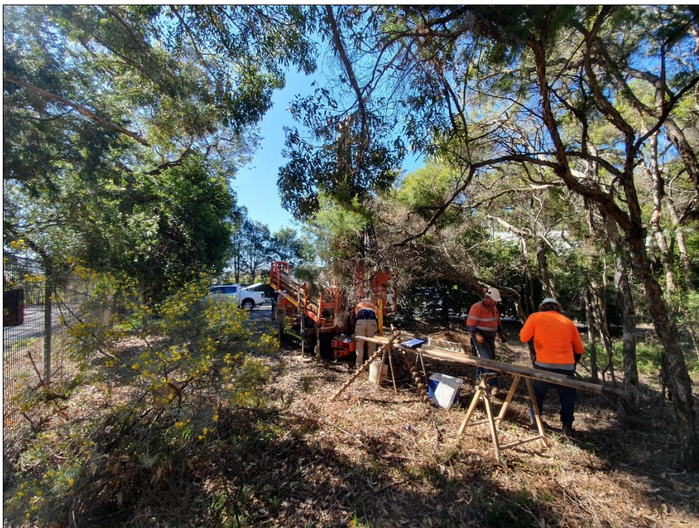
Photo 2 – AG's Site Investigation – Drilling BH102
