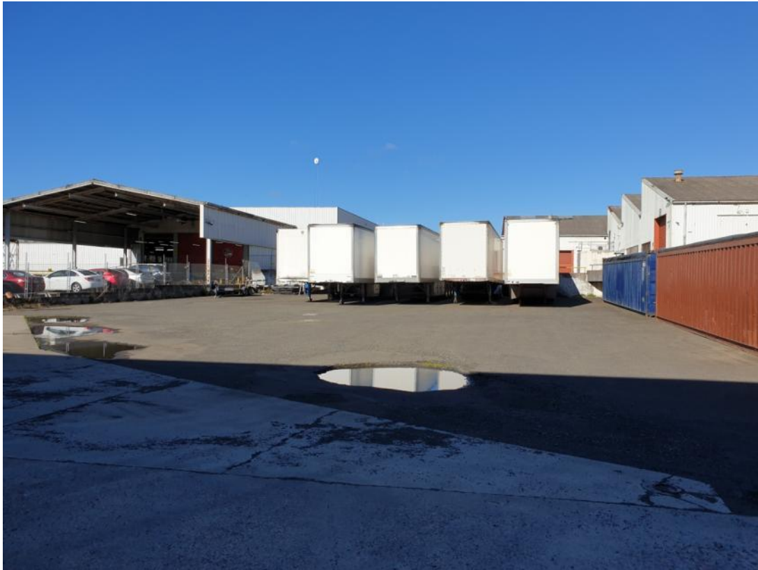
Figure 4.5 South-facing view showing the loading zone within the central portion of the study area and the two-storey warehouse buildings to the right.
