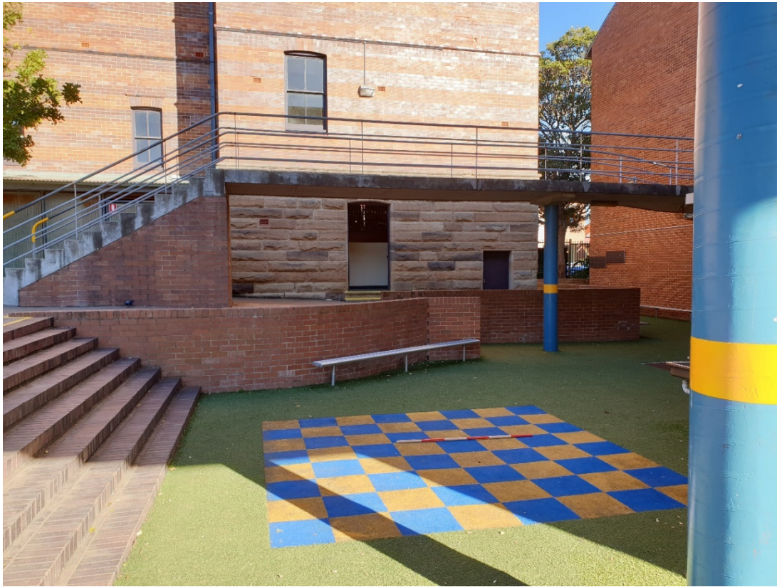
Figure 4.6 View to the south with buildings A (centre) and building E (to the right), the level of earthworks can be seen clearly as the ground level building A was constructed on is approximately 0.5m above the level building E was constructed on.
