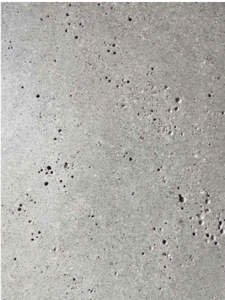
CONCRETE BLEACHERS LIGHTLY EXPOSED CONCRETE. FINISH TO COMPLY WITH P5 SLIP RATING FOR STEPS AND RAMPS.
