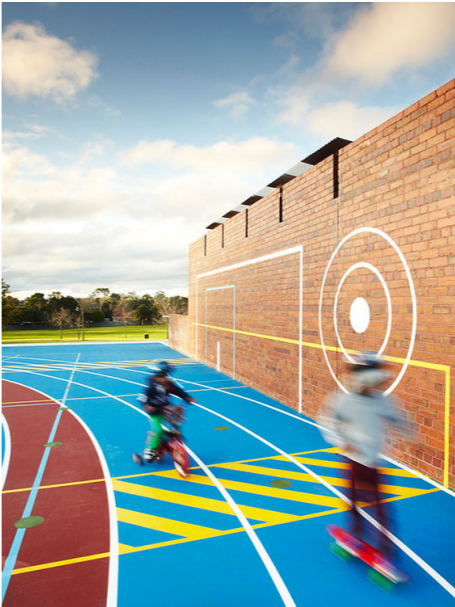
MULTI COURT PAINTED SURFACE FOR BALL GAMES. FINISH TO COMPLY WITH P4 SLIP RATING FOR GENERAL PAVEMENT, P5 FOR STEPS AND RAMPS.
