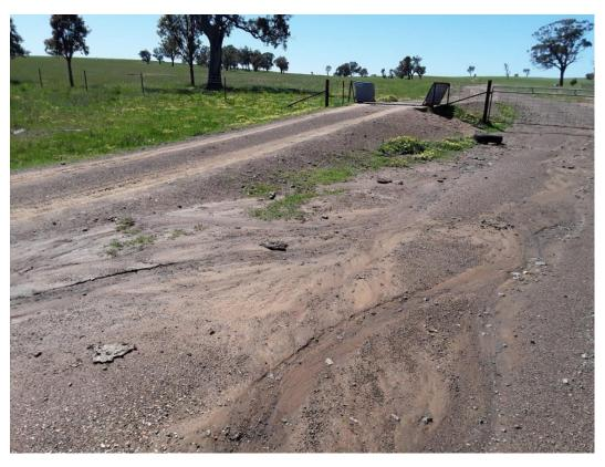
Photo 9-5: Washout and drainage rills on road and adjacent track, on unvegetated soils in the north east of the study area
