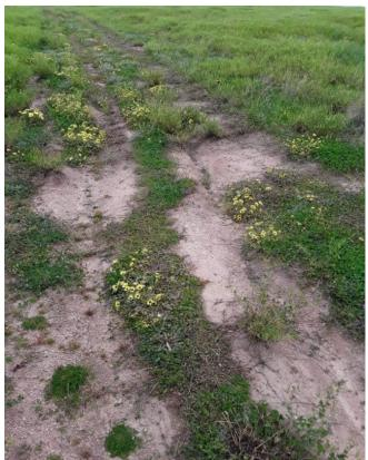
Photo 9-4: Minor drainage rills on track, on unvegetated area slope 4-5 per cent, in the north west of the study area
