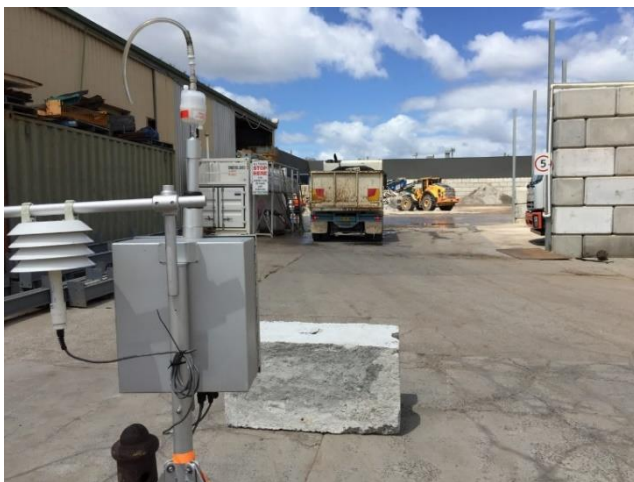
Figure 2 AQ monitoring station (looking south)
