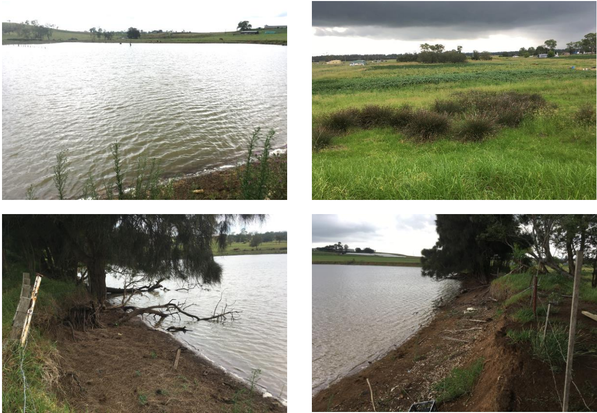
Figure 16: Photo point 8: Top left: looking upstream across 6 th dam; top right: looking downstream from 6 th dam; bottom left and right: dam wall erosion and C. glauca trees.
