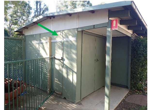
Photo 24: Shed, non-asbestos containing fibre cement sheeting to the external walls
