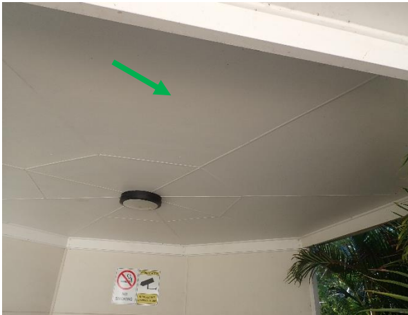
Photo 22: Gazebo, non-asbestos containing fibre cement sheeting to the ceiling
