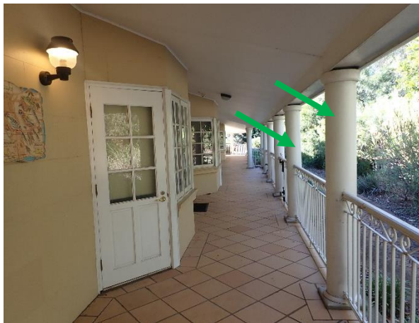
Photo 4: Lodge, non-asbestos containing moulded fibre cement columns to veranda
