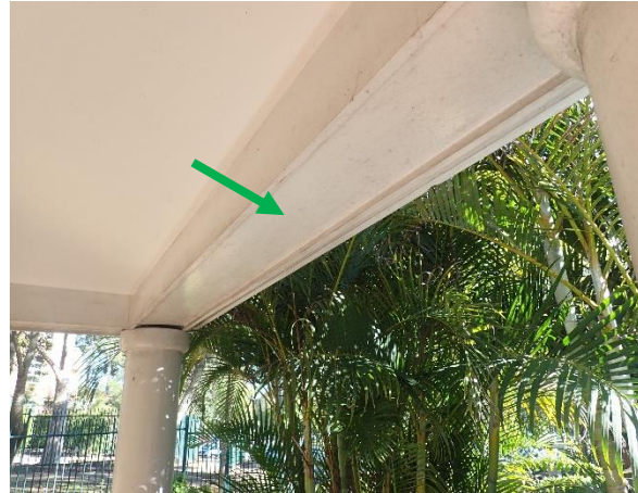
Photo 2: Lodge, non-asbestos containing fibre cement sheeting to eaves
