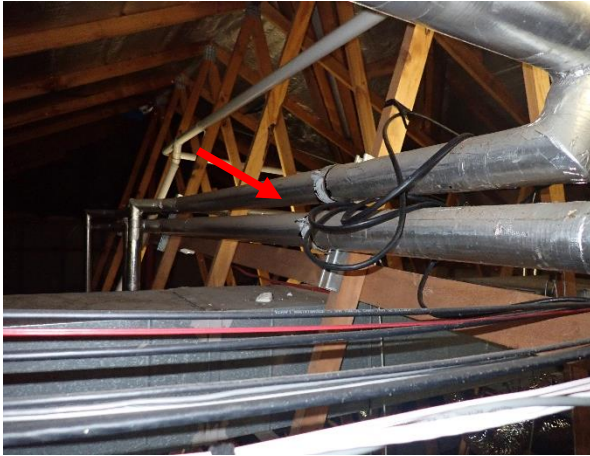
Photo 19: Lodge, assumed SMF insulation to pipework throughout ceiling cavity
