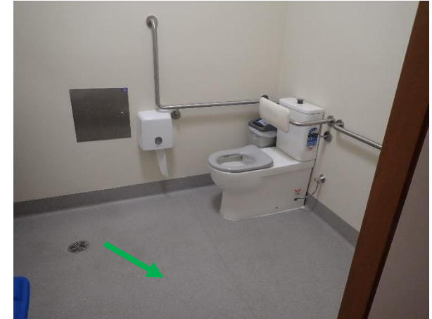
Photo 9: Lodge, non-asbestos containing grey vinyl flooring to east disabled toilet
