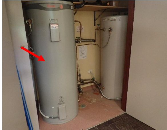
Photo 14: Lodge, assumed internal SMF insulation to hot water systems in east HWS cupboard
