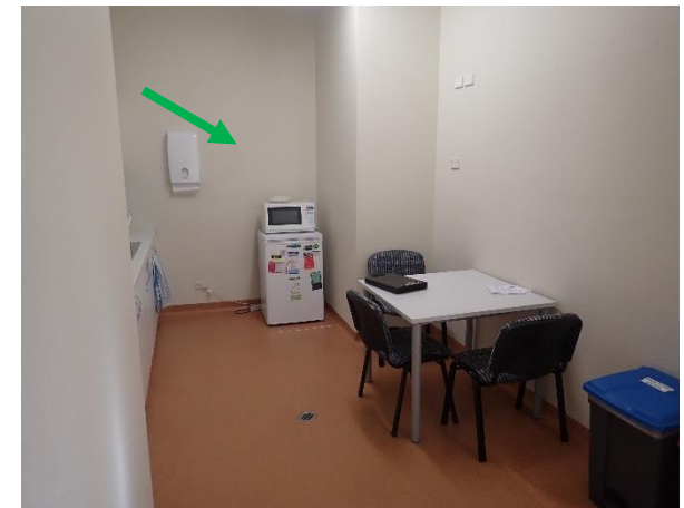
Photo 6: Lodge, non-asbestos containing fibre cement sheeting to east kitchen walls
