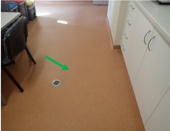
Photo 7: Lodge, non-asbestos containing brown vinyl flooring to east kitchen
