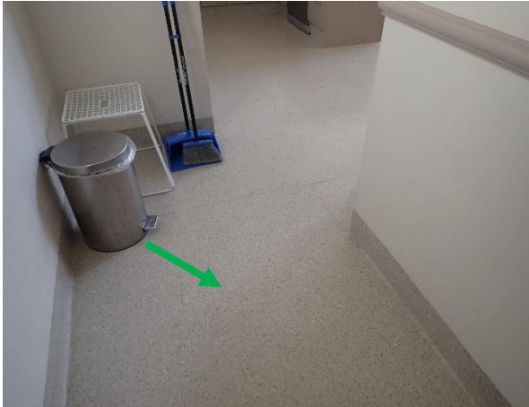
Photo 13: Lodge, non-asbestos containing grey vinyl flooring to E1 kitchen
