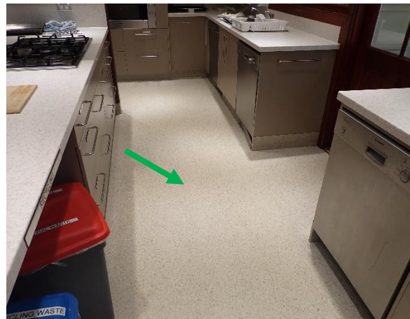
Photo 11: Lodge, non-asbestos containing grey vinyl flooring to central kitchen
