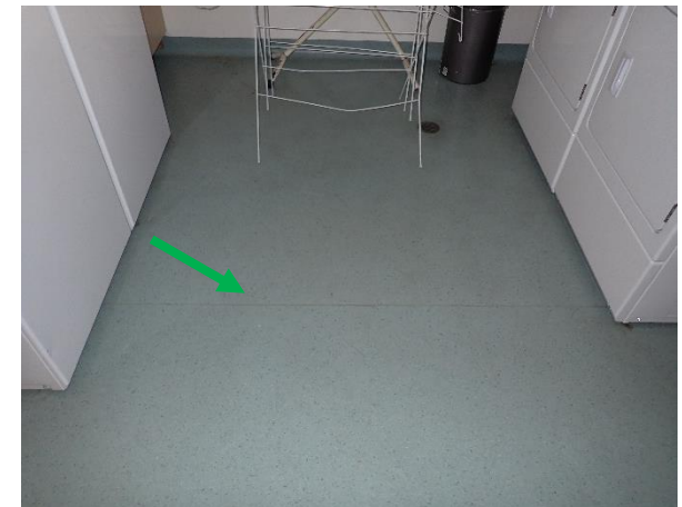
Photo 12: Lodge, non-asbestos containing green vinyl flooring to west laundry
