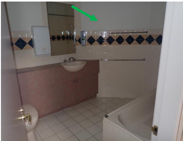
Photo 10: Lodge, non-asbestos containing fibre cement sheeting to bathroom walls throughout
