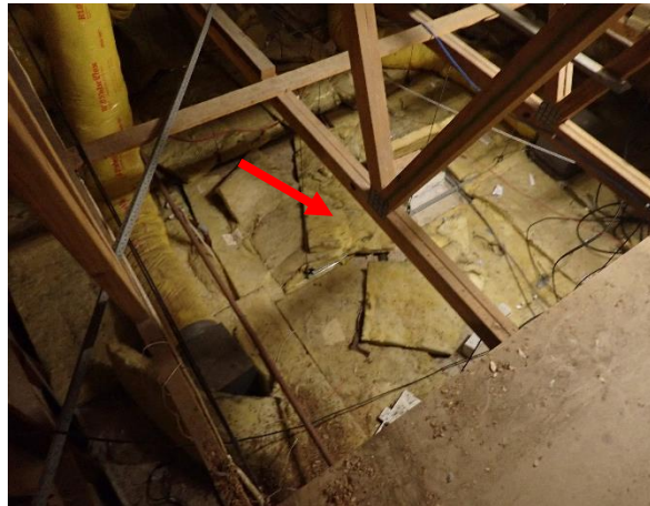
Photo 17: Lodge, assumed SMF insulation batts throughout the ceiling cavity
