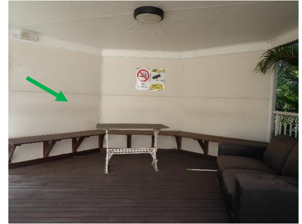
Photo 21: Gazebo, non-asbestos containing fibre cement sheeting to the north wall
