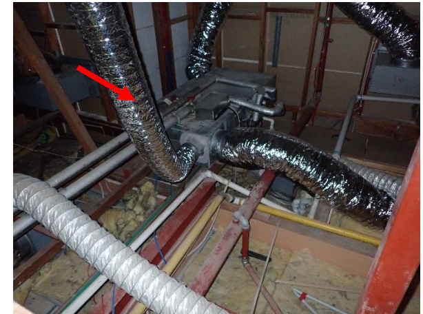
Photo 18: Lodge, assumed SMF insulation to air conditioning ducting throughout ceiling cavity
