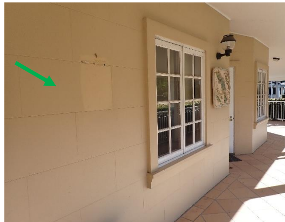
Photo 5: Lodge, non-asbestos containing fibre cement sheeting to external walls
