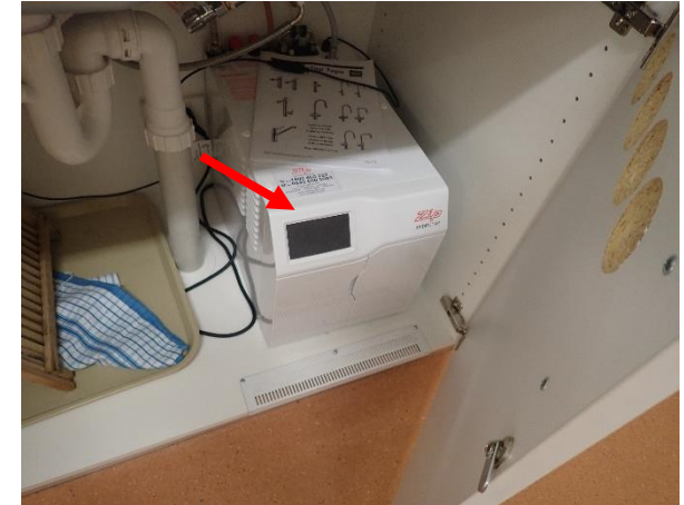
Photo 15: Lodge, assumed internal SMF insulation to instant hot/cold water system in east kitchen
