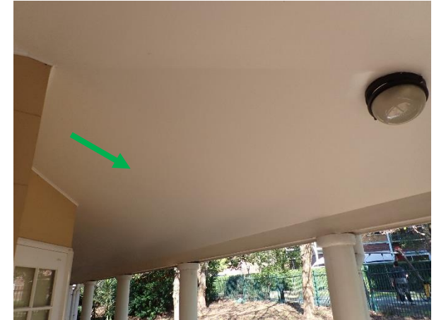
Photo 3: Lodge, non-asbestos containing fibre cement sheeting to veranda soffits
