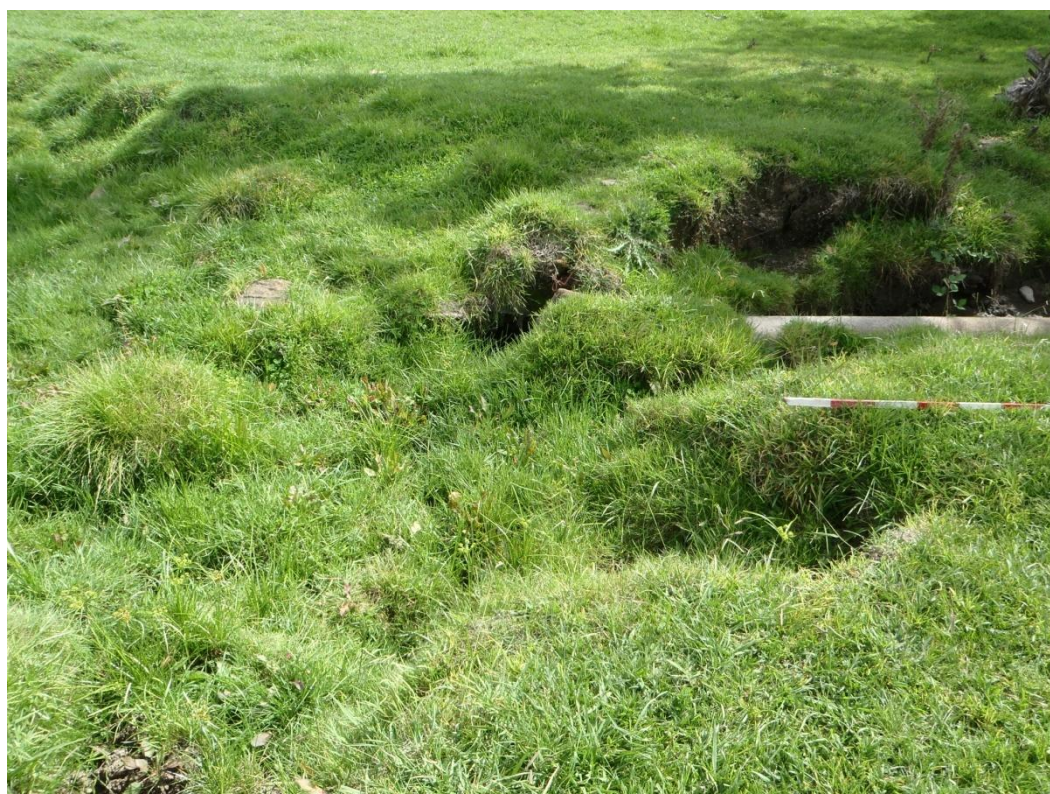
Photo 3. The breach at the upstream end of the farm dam where Stony Creek flows out of the dam pond. Site C on Figure 1. The scale pole is 1.5m long with 15cm divisions.
