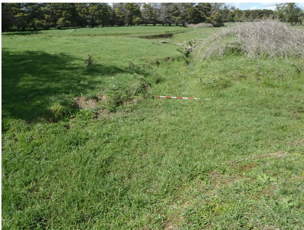
Photo 3. The breach at the upstream end of the farm dam where Stony Creek flows out of the dam pond. Site C on Figure 1. The scale pole is 1.5m long with 15cm divisions.
