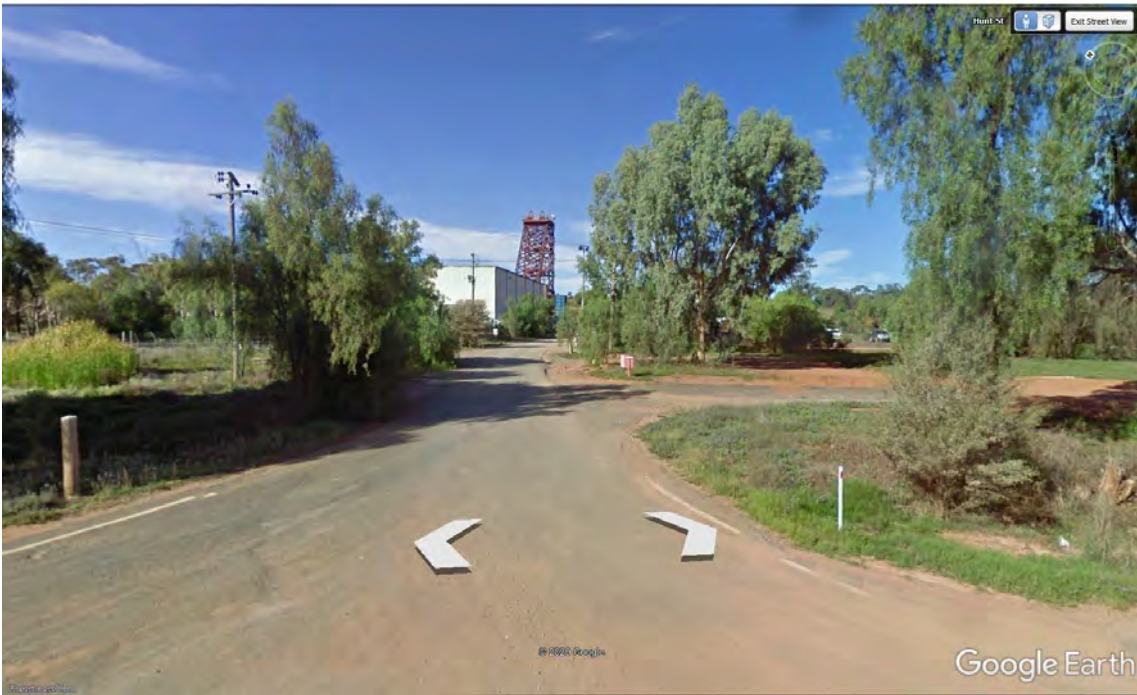
Plate 5.10 New Cobar Complex mine industrial area (Source: Google street view)
