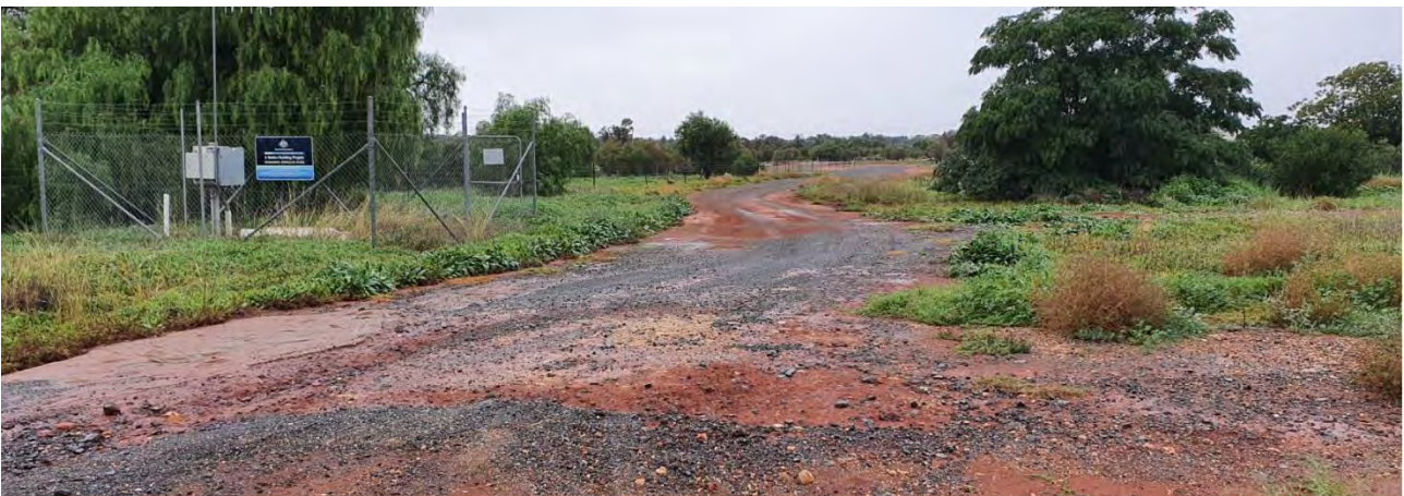
Plate 2.10 Power line construction vehicular access road
