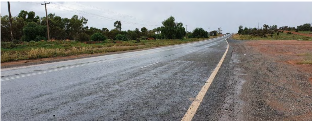
Plate 2.5 Localised widening and sight distance to the south along Kidman Way at New Cobar Complex
