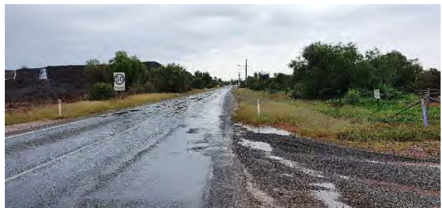
Looking right from site access (470 m)
