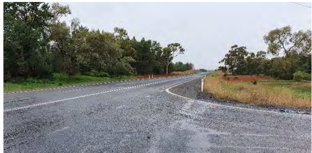
Looking right from site access (330 m)
