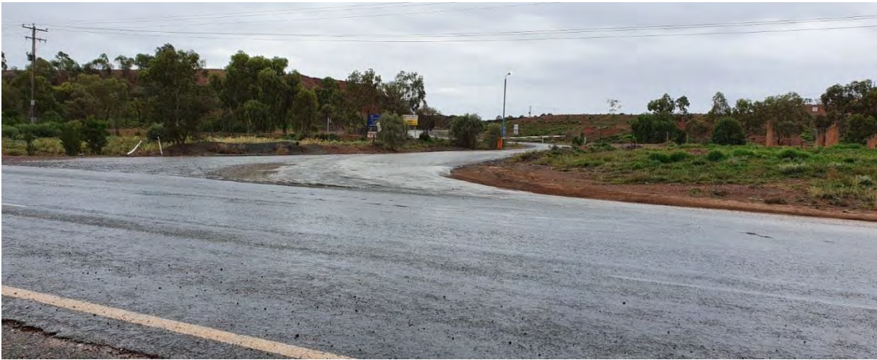
Plate 2.4 Kidman Way/ New Cobar Complex intersection (view east)
