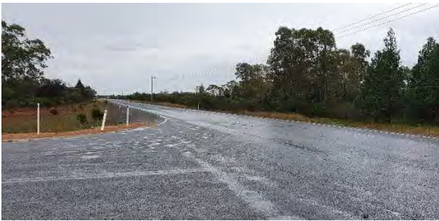
Looking left from site access (295 m)
